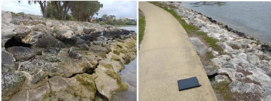
**Figure 3.12 Grouted Revetment (L) & Voids Under Path (R)**
