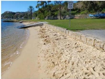
**Figure 3.35 Limestone Blockwall**
