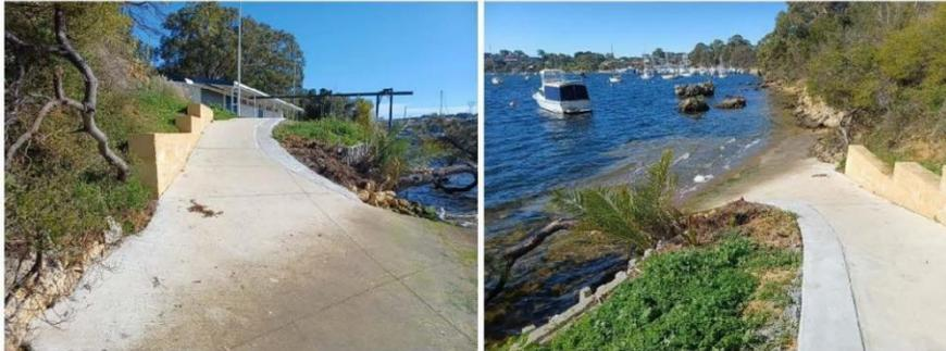
**Figure 3.25 Limestone Block Wall & Concrete Apron**
