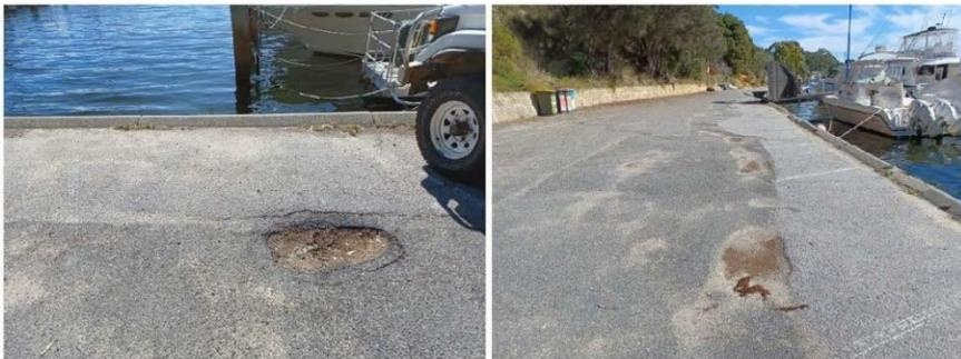
**Figure 3.29 Carpark Pot Holes & Repairs**
