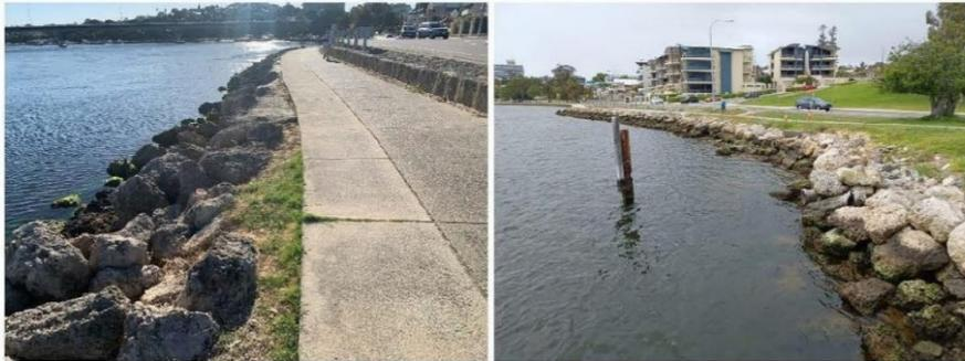
**Figure 3.1 Path Behind Revetment (L) & Overtopping Damage (R)**
