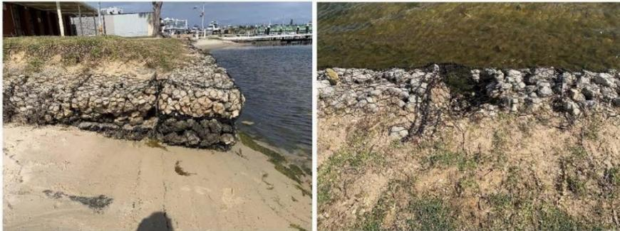
**Figure 3.18 Limestone Gabions Rotated (L) & Lost Material (R)**
