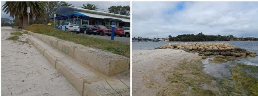
**Figure 3.14 Block Wall (L) & Groyne Example (R)**
