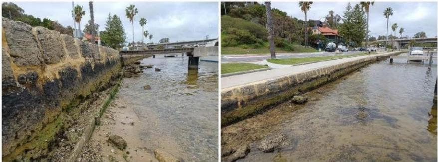
**Figure 3.5 Limestone Blockwall with Jetty Abutments**
