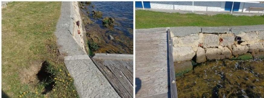
**Figure 3.23 Deteriorated Limestone Block Wall**
