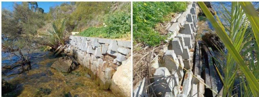
**Figure 3.24 Deteriorated Crib Wall**
