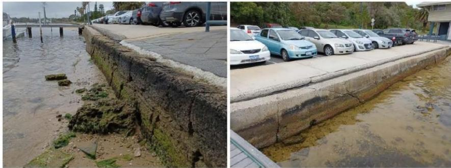
**Figure 3.7 Weathered Blockwall (L) & Cracking of Concrete Wall (R)**
