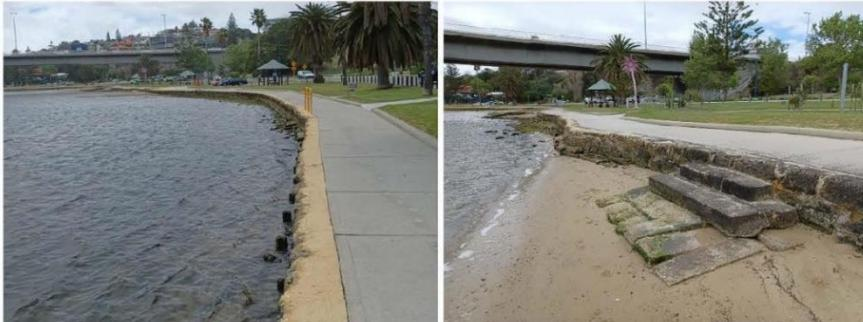
**Figure 3.3 Limestone Block Wall (L) & Access Stairs (R)**
