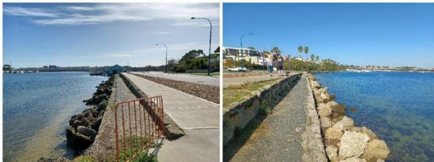
**Figure 3.9a Limestone Armour in Front of Vertical Wall**
