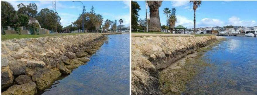
**Figure 3.22 Pitched Limestone Revetment**
