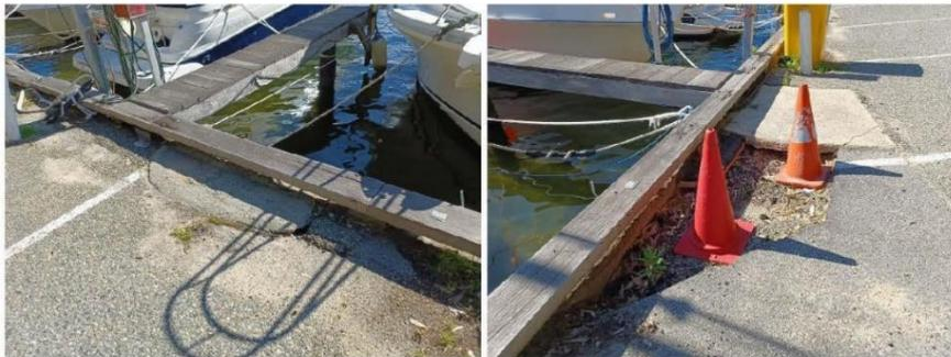
**Figure 3.31 Carpark Bitumen Repairs & Settlement**
