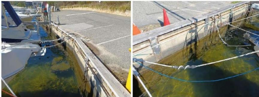
**Figure 3.30 Concrete Panel & Steel Pile Wall**
