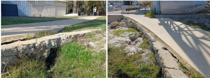
**Figure 3.21 Undermined Limestone Block Wall**
