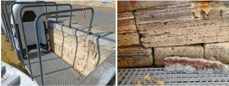
**Figure 3.32 Limestone Blockwall with Dinghy Rack**
