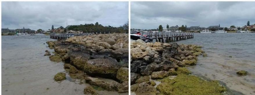
**Figure 3.13 Revetment Around Boat Ramp**
