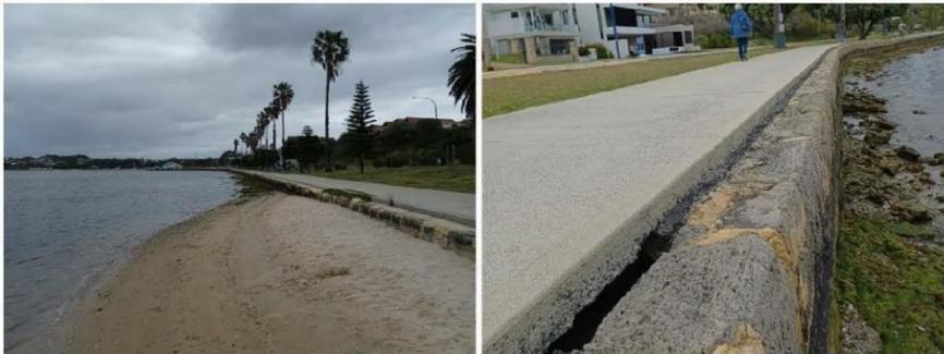
**Figure 3.8 Low Limestone Blockwall (L) & Voids Beneath Path (R)**
