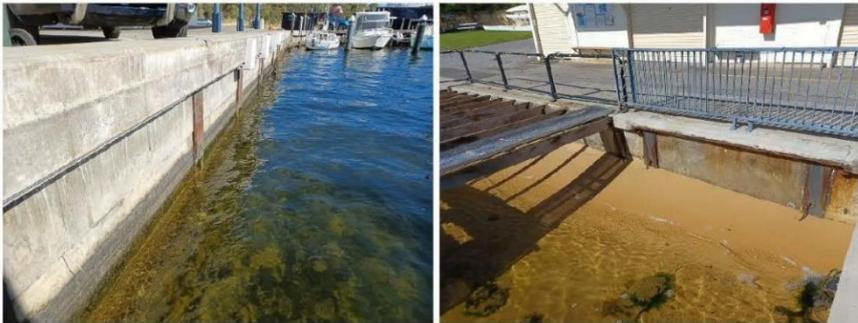
**Figure 3.34 Concrete Panel & Steel H-Pile Wall**
