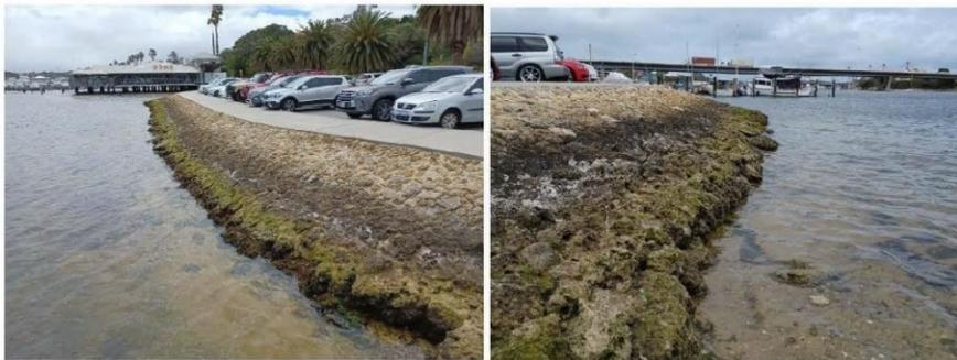
**Figure 3.6 Pitched Revetment Looking North (L) & South (R)**
