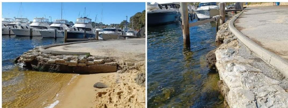
Figure 3.27 Grout Filled Bags
