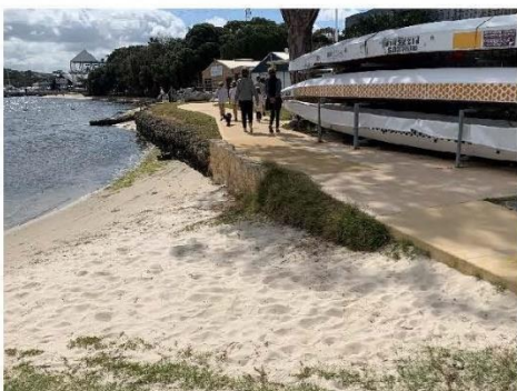
Figure 3.17 Limestone Block Wall
