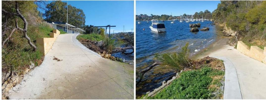
Figure 3.25 Limestone Block Wall & Concrete Apron
