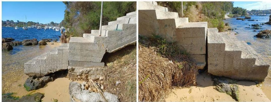
Figure 3.26 Concrete Stair Abutment
