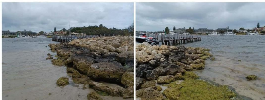
Figure 3.13 Revetment Around Boat Ramp
