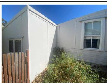
Figure 4: Existing addition to rear of cottage to be removed, element 2022
