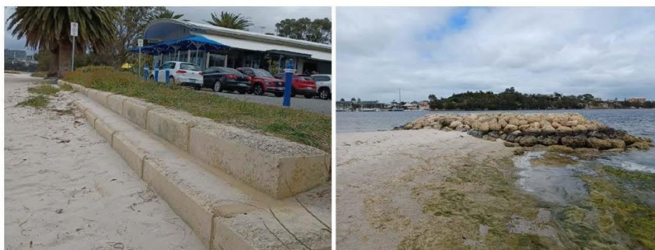
Figure 3.14 Block Wall (L) & Groyne Example (R)
