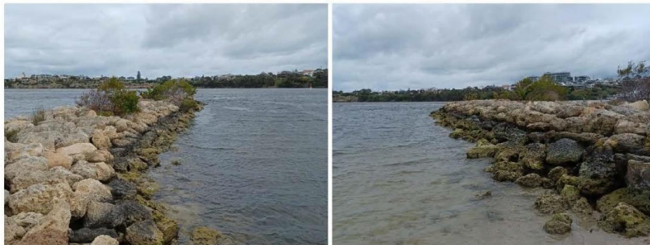
Figure 3.16 Preston Point Groyne
