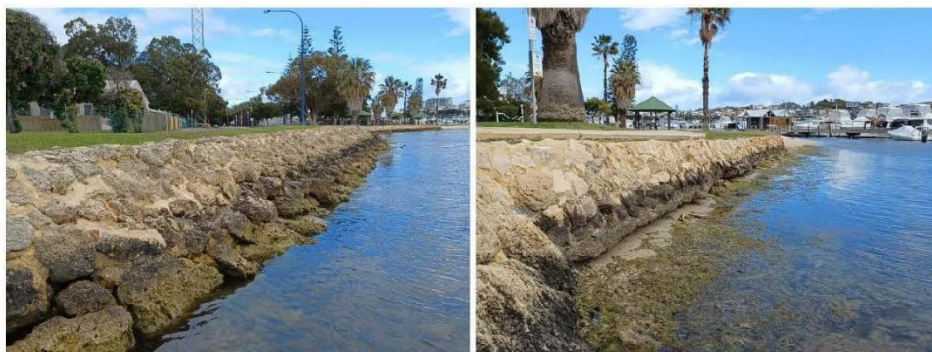
Figure 3.22 Pitched Limestone Revetment
