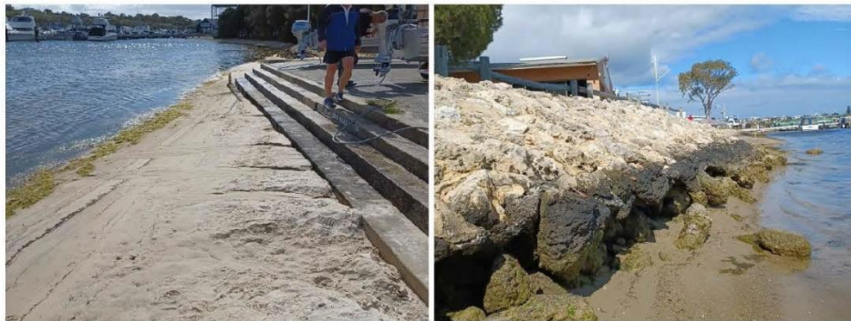
Figure 3.20 Steps (L) & Pitched Revetment (R)
