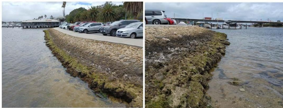
Figure 3.6 Pitched Revetment Looking North (L) & South (R)
