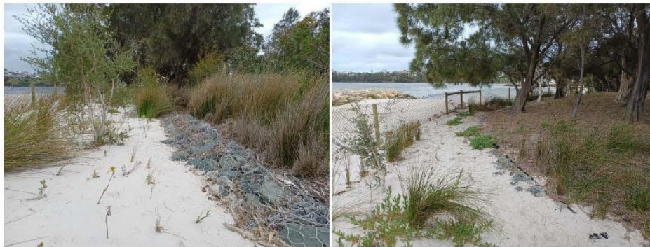
Figure 3.15 Buried Gabion/Reno Mattresses
