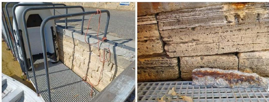
Figure 3.32 Limestone Blockwall with Dinghy Rack
