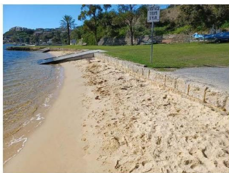
Figure 3.35 Limestone Blockwall
