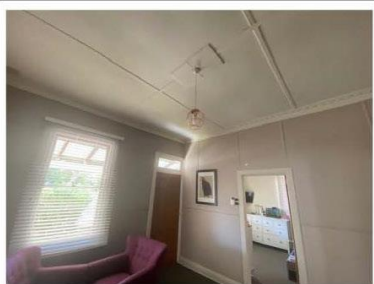
Figure 6: Internal doors to be modified, element 2022
