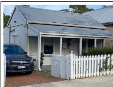
Figure 3: Existing street view, element 2022
