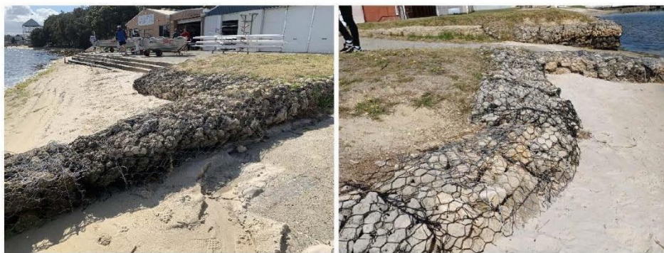
Figure 3.19 Limestone Gabions
