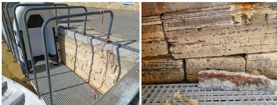
Figure 3.32 Limestone Blockwall with Dinghy Rack
