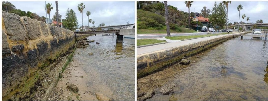
Figure 3.5 Limestone Blockwall with Jetty Abutments
