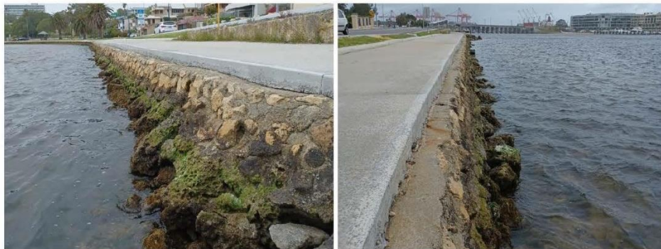
Figure 3.2 J Dolan Park Wall Looking East (L) & Looking West (R)
