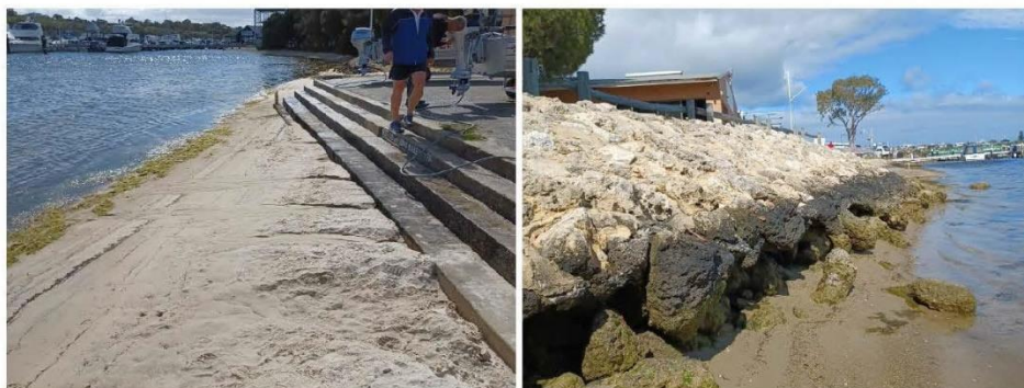
Figure 3.20 Steps (L) & Pitched Revetment (R)
