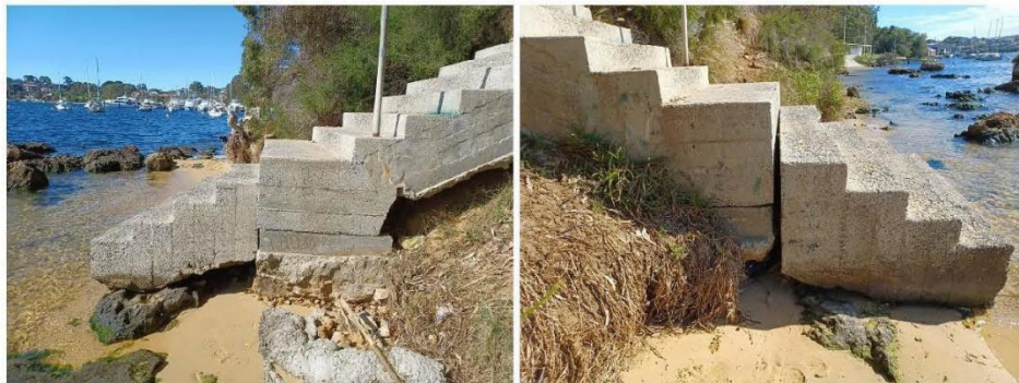
Figure 3.26 Concrete Stair Abutment
