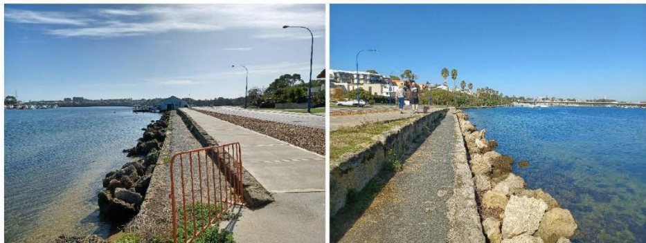
Figure 3.9a Limestone Armour in Front of Vertical Wall
