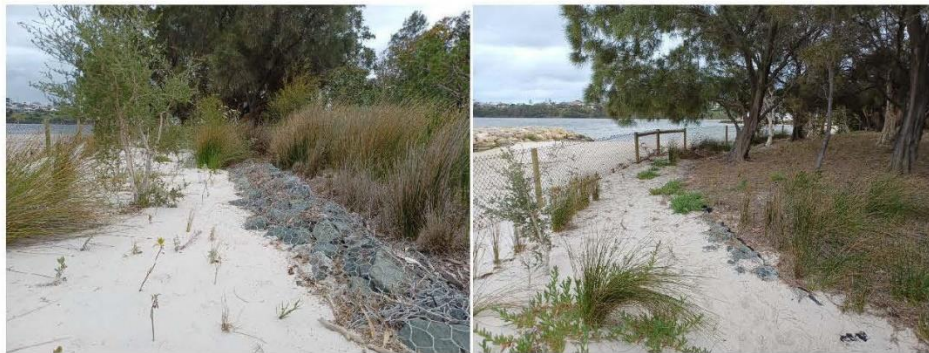
Figure 3.15 Buried Gabion/Reno Mattresses
