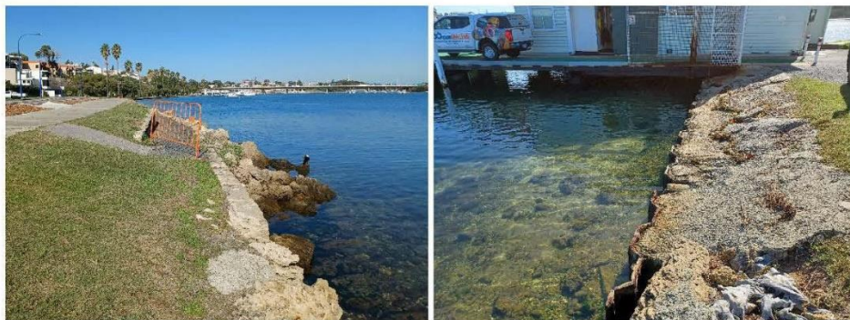
Figure 3.9b Tie In (L) & Sheet Pile Wall (R)
