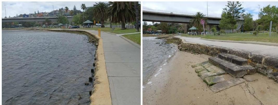
Figure 3.3 Limestone Block Wall (L) & Access Stairs (R)
