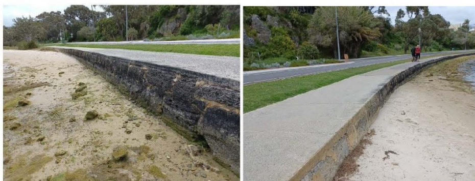
Figure 3.11 Limestone Block Wall & Sandy Beach
