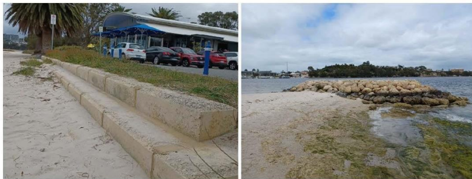
Figure 3.14 Block Wall (L) & Groyne Example (R)
