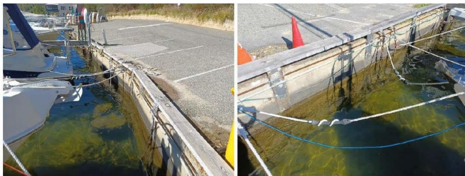
Figure 3.30 Concrete Panel & Steel Pile Wall
