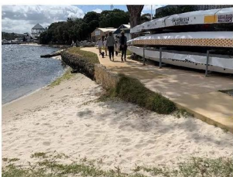
Figure 3.17 Limestone Block Wall
