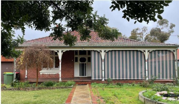
Photograph 1 View from the street. Griffiths Architects July 2022
