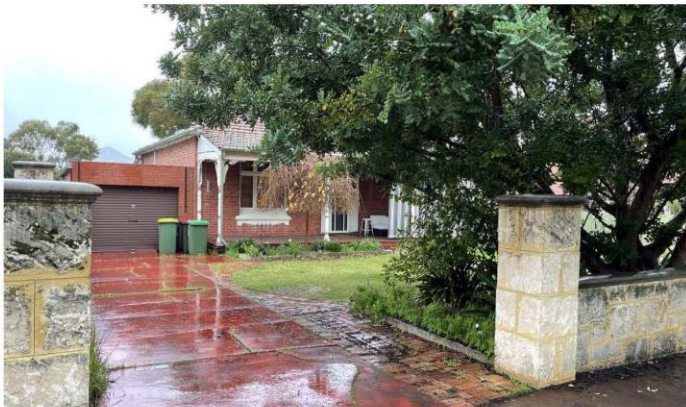
Photograph 2 Limestone fence and garage addition. Griffiths Architects July 2022
