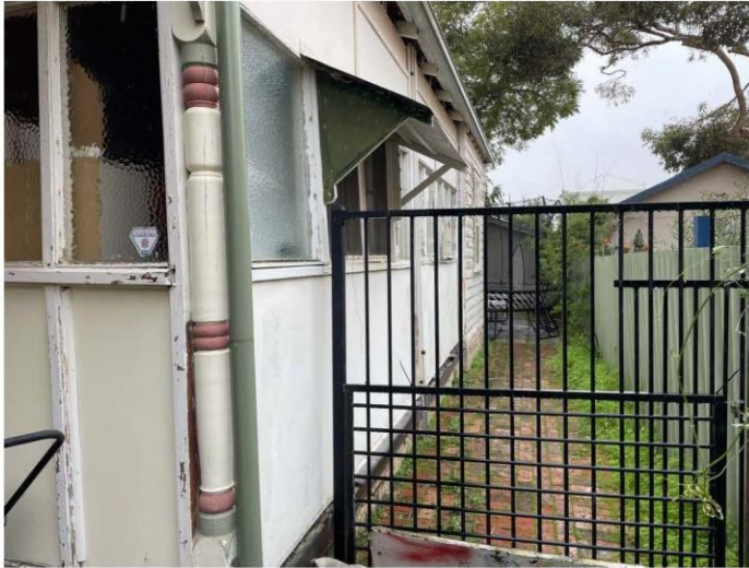
Photograph 4 The early timber addition to the rear and the more recent one in the foreground. Griffiths Architects July 2022 Some verandah posts remain and others may be concealed by the cladding.
