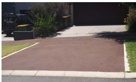
Image 1. Image shows red asphalt footpath and crossover.
