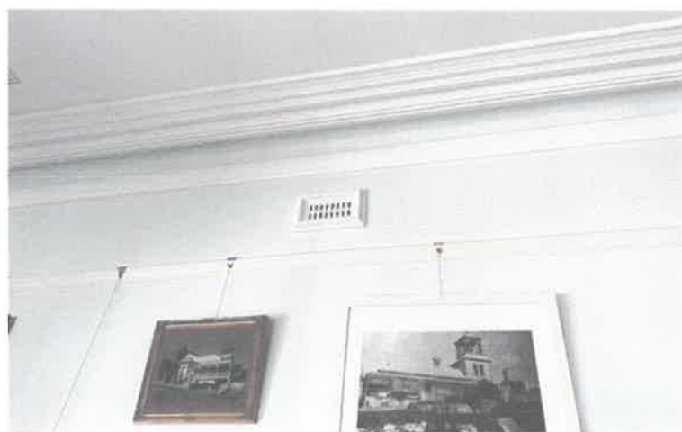
Original Cornices, Picture rails and Vents
