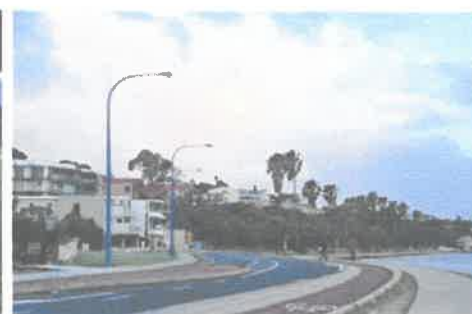
VIEW FROM Boat Shed Education; to the North (East Fremantle side of the river) The belvedere can only just be made out to the left of the palm trees in the foreground. It is our position that the change in the centre of the roof will not change this view in any perceptible way.
