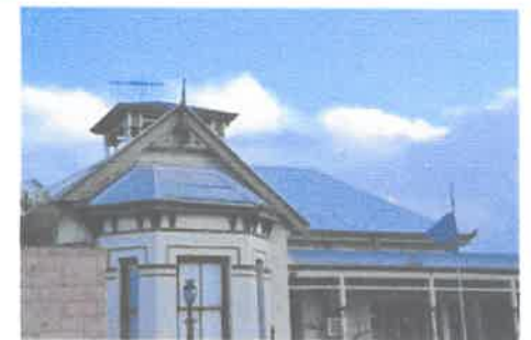
VIEW FROM 9 BOLTON STREET
