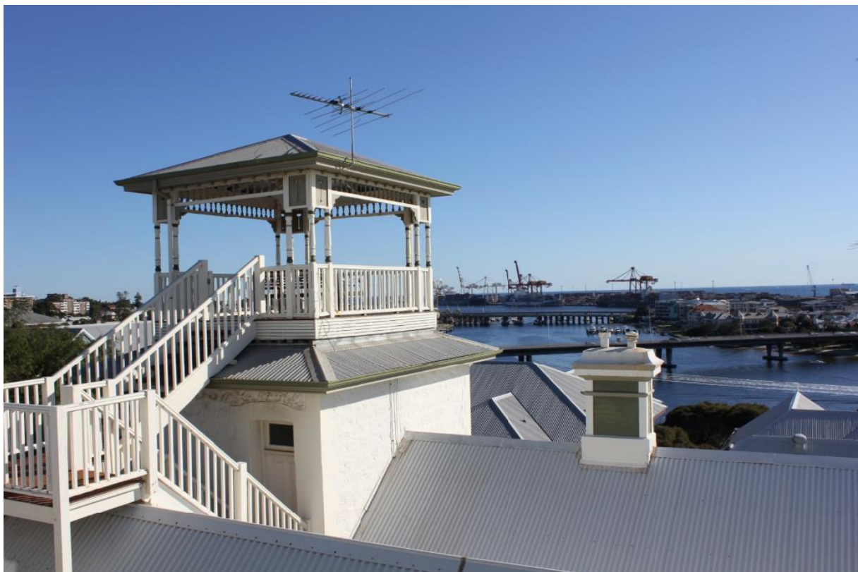
Figure 5. Roofline 10 Bolton Street.
