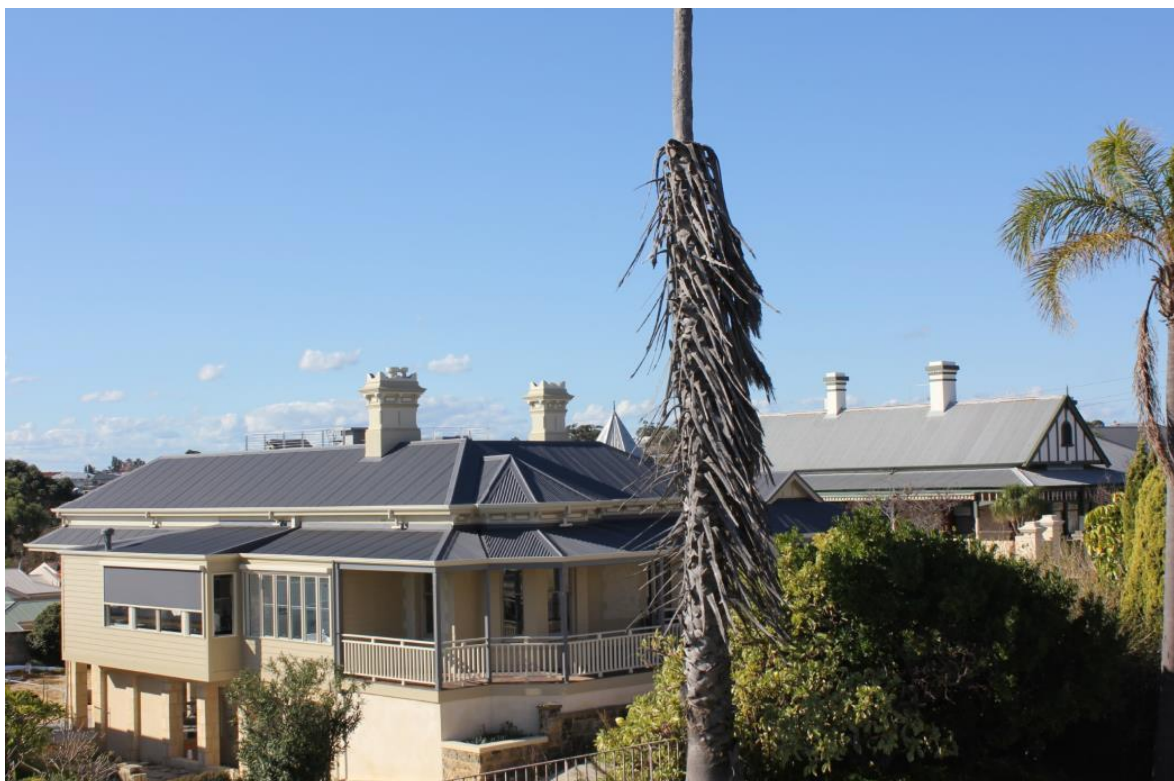
Figure 3. Roof line of 3 & 5 Bolton Street. Both show clear prominence of decorative chimneys and in the case of No. 5 significant renovation has taken place without diminishing traditional design.
