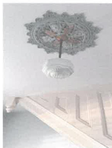
timber panelling and trims to existing stairwell
