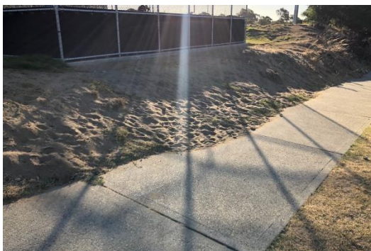
Sand on pathways – needs treatment to retain
