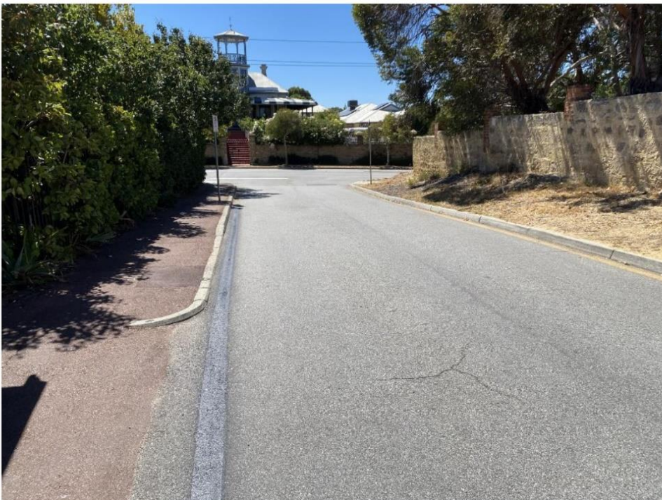
Bolton Street (looking east towards Preston Point Road)
