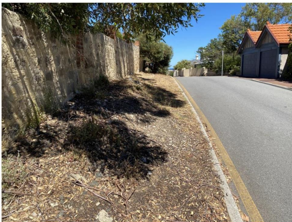
Steep and narrow verge with high retaining on southern side
