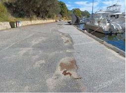
Figure 3.29 Carpark Pot Holes & Repairs
