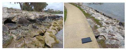
Figure 3.12 Grouted Revetment (L) & Voids Under Path (R)
