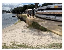
Figure 3.17 Limestone Block Wall
