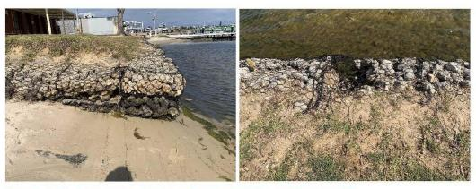
Figure 3.18 Limestone Gabions Rotated (L) & Lost Material (R)
