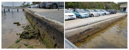
Weathered Blockwall (L) & Cracking of Concrete Wall (R)
