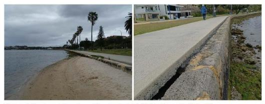
Figure 3.8 Low Limestone Blockwall (L) & Voids Beneath Path (R)
