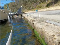
Figure 3.28 Limestone Blockwall
