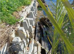
Figure 3.24 Deteriorated Crib Wall
