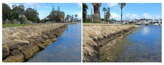
Figure 3.22 Pitched Limestone Revetment
