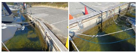
Figure 3.30 Concrete Panel & Steel Pile Wall
