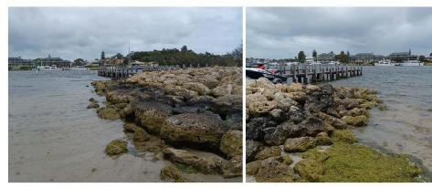
Figure 3.13 Revetment Around Boat Ramp
