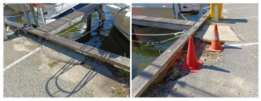
Figure 3.31 Carpark Bitumen Repairs & Settlement
