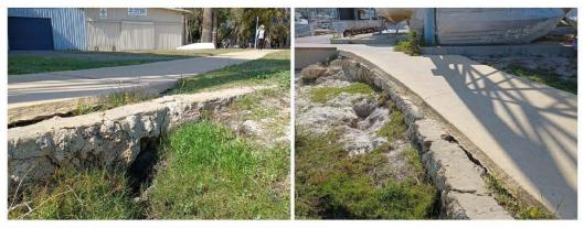
Figure 3.21 Undermined Limestone Block Wall
