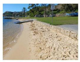
Figure 3.35 Limestone Blockwall
