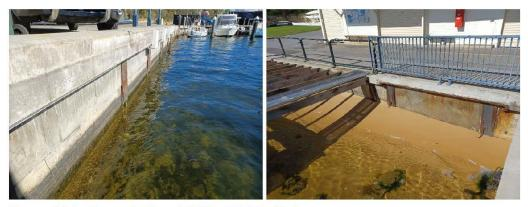
Figure 3.34 Concrete Panel & Steel H-Pile Wall
