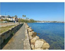
Figure 3.9a Limestone Armour in Front of Vertical Wall
