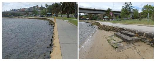
Figure 3.3 Limestone Block Wall (L) & Access Stairs (R)
