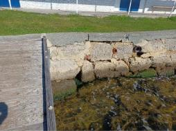
Figure 3.23 Deteriorated Limestone Block Wall
