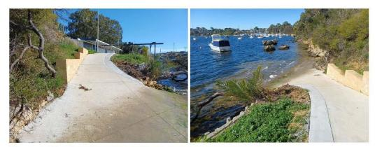
Figure 3.25 Limestone Block Wall & Concrete Apron
