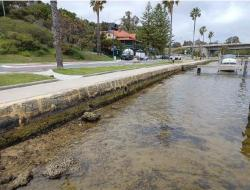
Figure 3.5 **Limestone Blockwall with Jetty Abutments**
