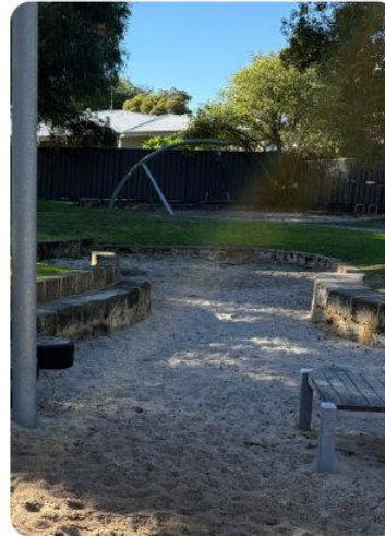
Existing limestone retaining wall
