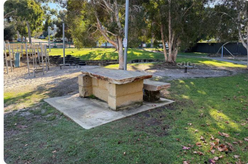
Existing site condition
