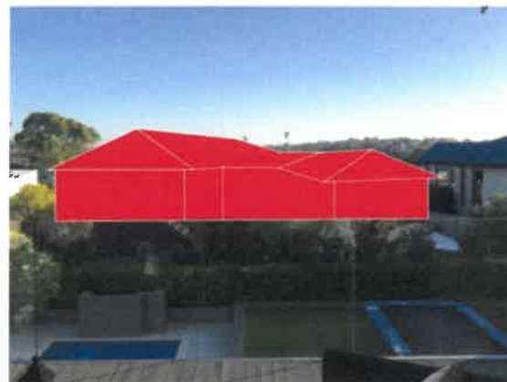
152 preston point rd # 152 Preston Point Road with potential compliant first floor addition, approximately 5.6m plate heights and 8.1m ridge height
