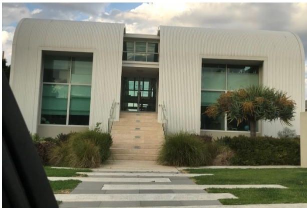
No. 10 Habgood Street, East Fremantle.
