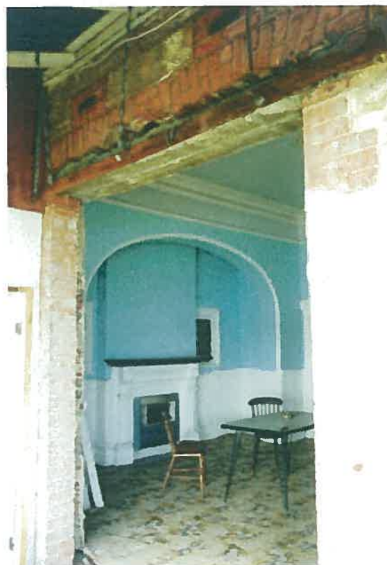
Missing wall and window to front elevation implemented c.1950s
