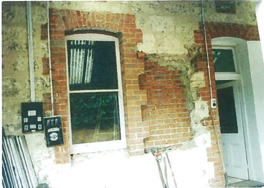
Repositioning of window to rear elevation 1987
