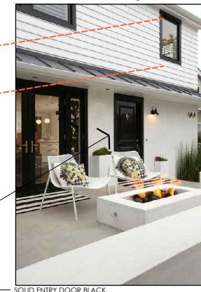
SOLID ENTRY DOOR BLACK ALL OTHER WINDOWS AND DOORS TIMBER FRAMED PAINTED VIVID WHITE
