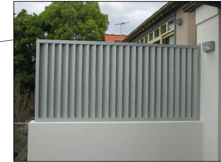
MINIMUM 1700mm HIGH BALCONY ALUMINIUM OR SIMILAR PRIVACY SCREEN - CAN BE A SOLID BRICK WALL OR FROSTED GLASS SCREEN MINIMUM 1.6m HIGH
