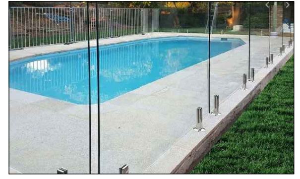
1200 HIGH GLASS POOL SAFETY FENCE AND GATE + EXTERNAL STAIRCASE GLASS BALUSTRADE + EXTERNAL BALCONY BALUSTRADE
