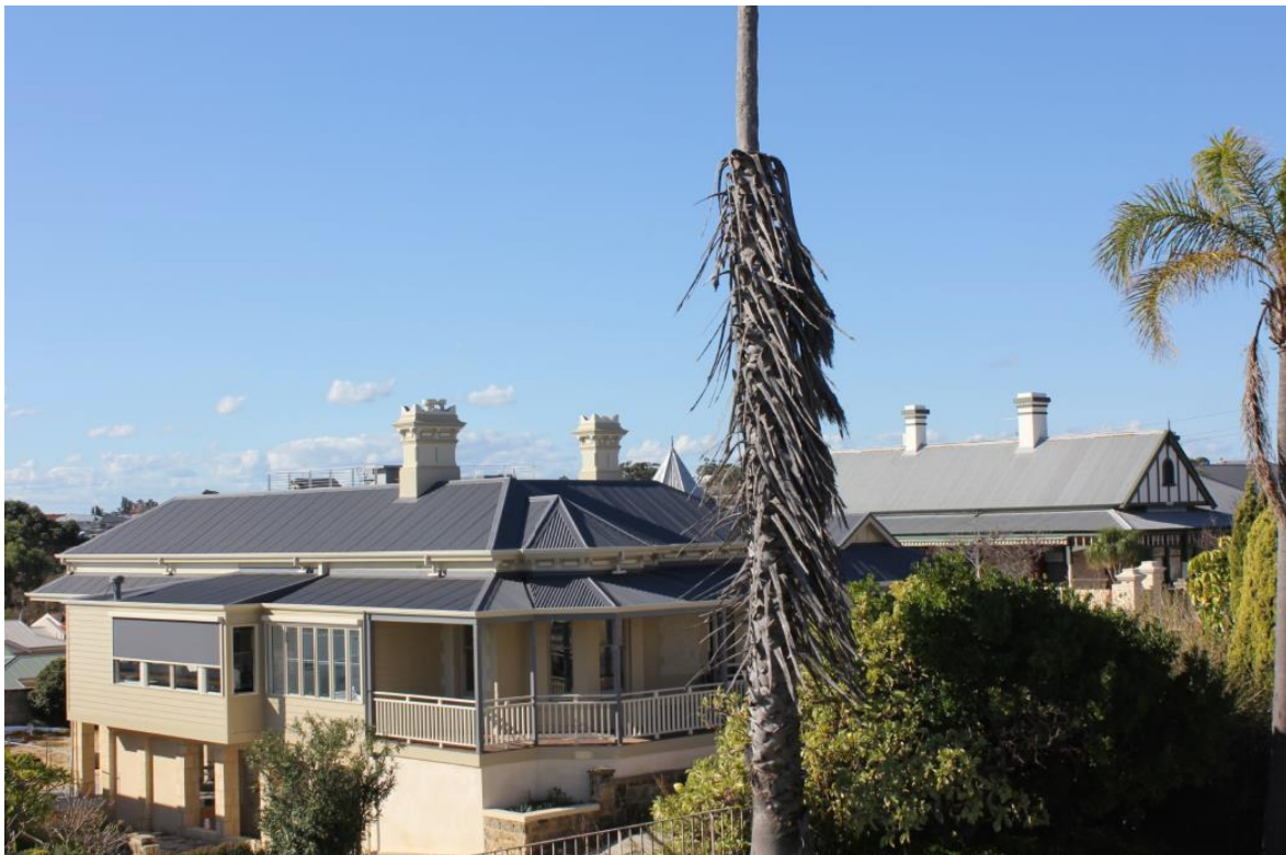
Figure 3. Roof line of 3 & 5 Bolton Street. Both show clear prominence of decorative chimneys and in the case of No. 5 significant renovation has taken place without diminishing traditional design.
