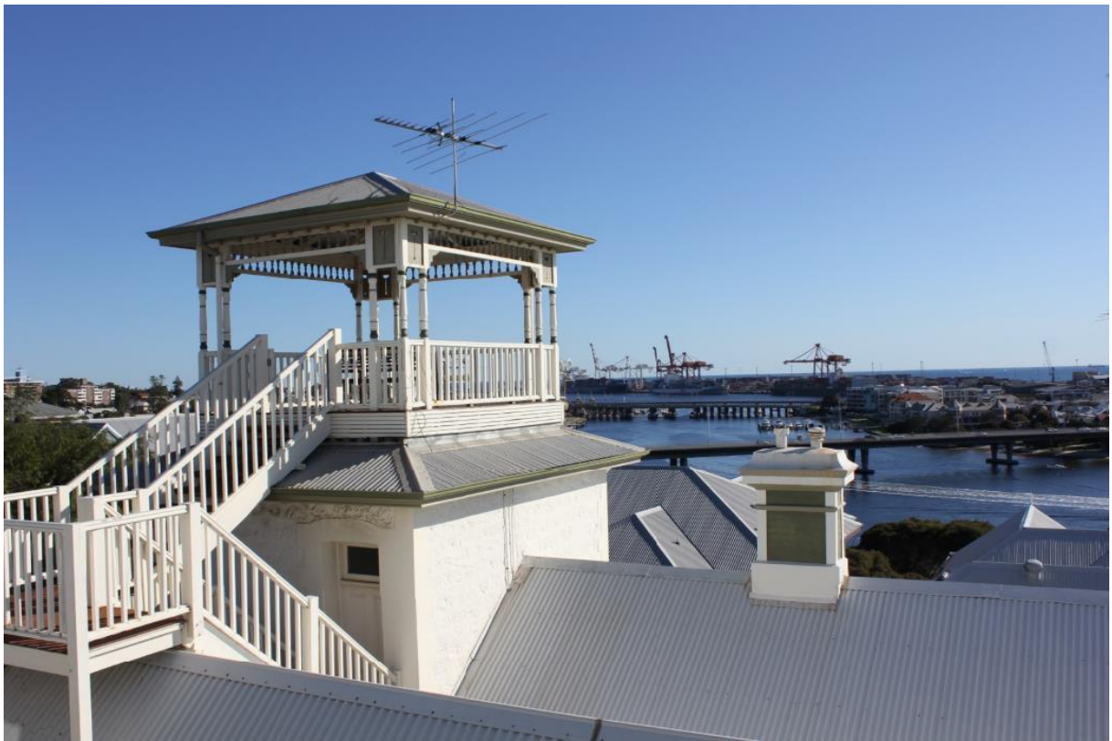
Figure 5. Roofline 10 Bolton Street.
