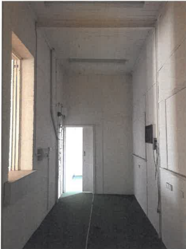
Image 10: Surface mounted conduits to be removed and consolidated, image taken by DPLH October 2017.
