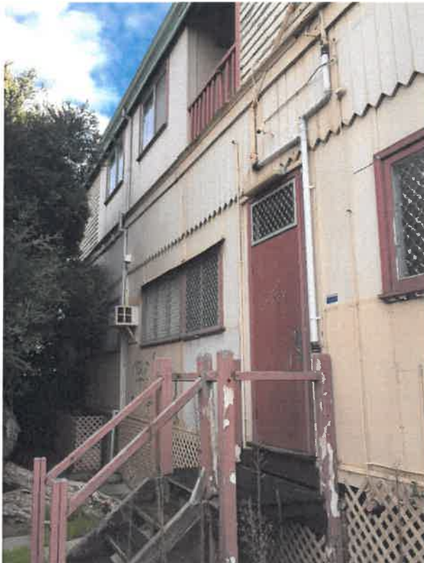
Image 6: Existing timber steps to be removed, image taken by DPLH October 2017.
