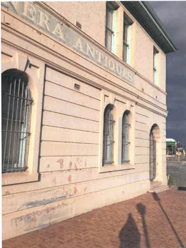
Image 8: Pavement to be cut back to allow for installation of breathing strip, image taken by DPLH October 2017.
