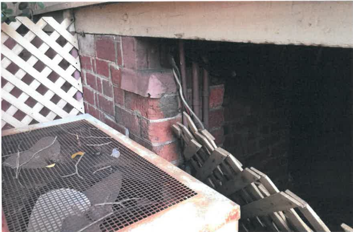
Image 7: Air conditioner unit to be removed, image taken by DPLH October 2017.
