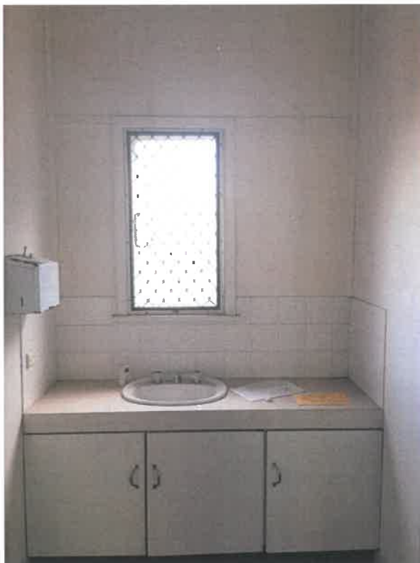
Image 16: WC bathroom cabinetry to be removed, image taken by DPLH October 2017.
