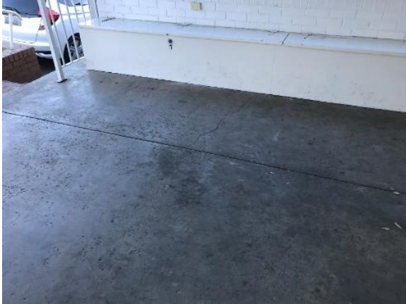
Photo 17-5-19, 8 49 32 am • Cracks in the concrete slab. Recommend investigating the cause of the crack. Rectification works can include patching the crack and painting the entire area.
