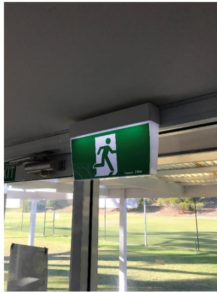
Photo 17-5-19, 8 53 37 am • Internal snib locks to exit doors do not comply with current requirements – these should be replaced with lever action locks / handles. • Illuminated exit sign is not in the correct location.
