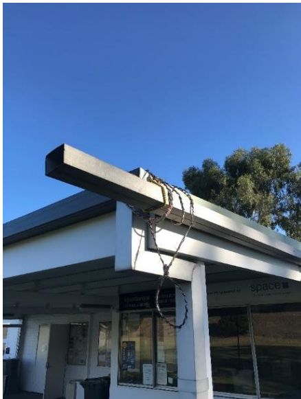
Photo 17-5-19, 8 50 01 am • Incomplete rain water pipe not securely fixed.
