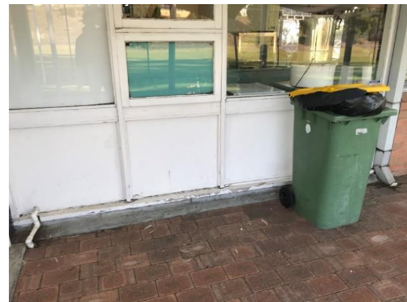
Photo 17-5-19, 8 50 30 am • Timber windows / doors to be stripped back (paint), puttied up, primed and painted.
