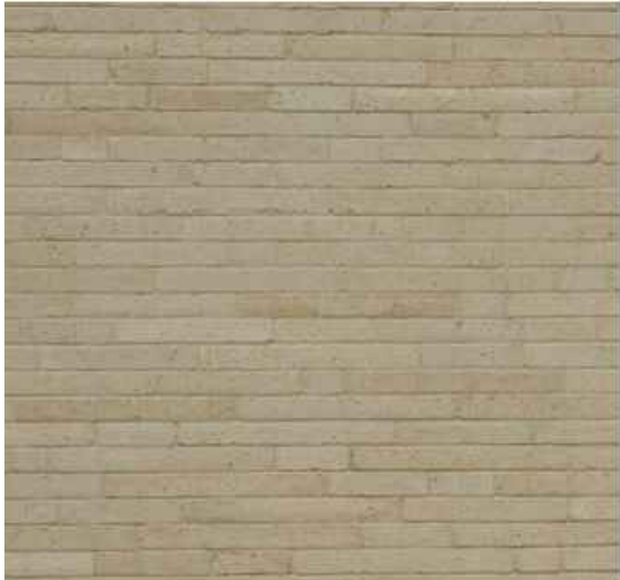
BR-01 EXPOSED BRICK WORK
