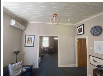
Figure 5: Internal wall to be removed, element 2022
