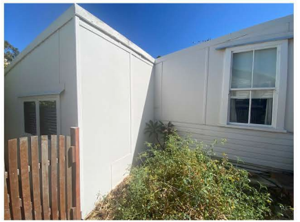
Figure 4: Existing addition to rear of cottage to be removed, element 2022
