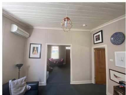
Figure 5: Internal wall to be removed, element 2022
