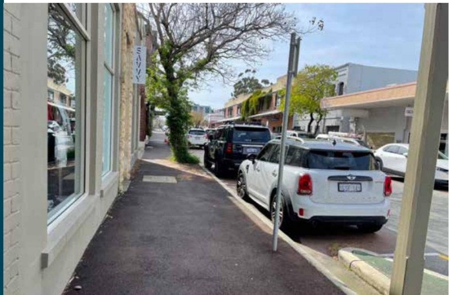
Upgraded footpaths on George Street
