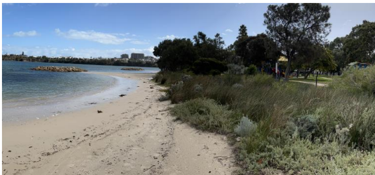
Figure 17.1: Example of nature-based stabilisation technique - revegetation of foreshore at John Tonkin Reserve shoreline
