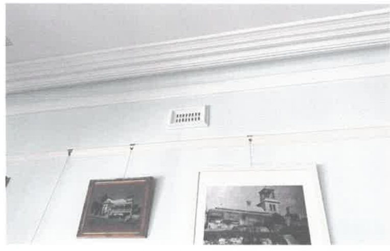
Original Cornices, Picture rails and Vents
