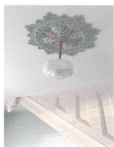
timber panelling and trims to existing stairwell
