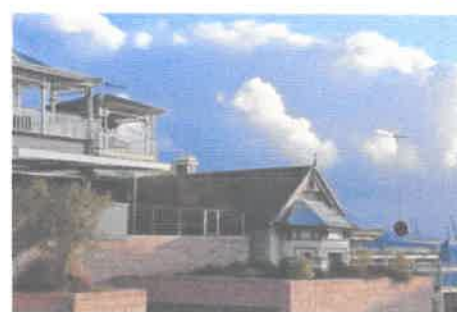
VIEW FROM 7 Bolton Street
