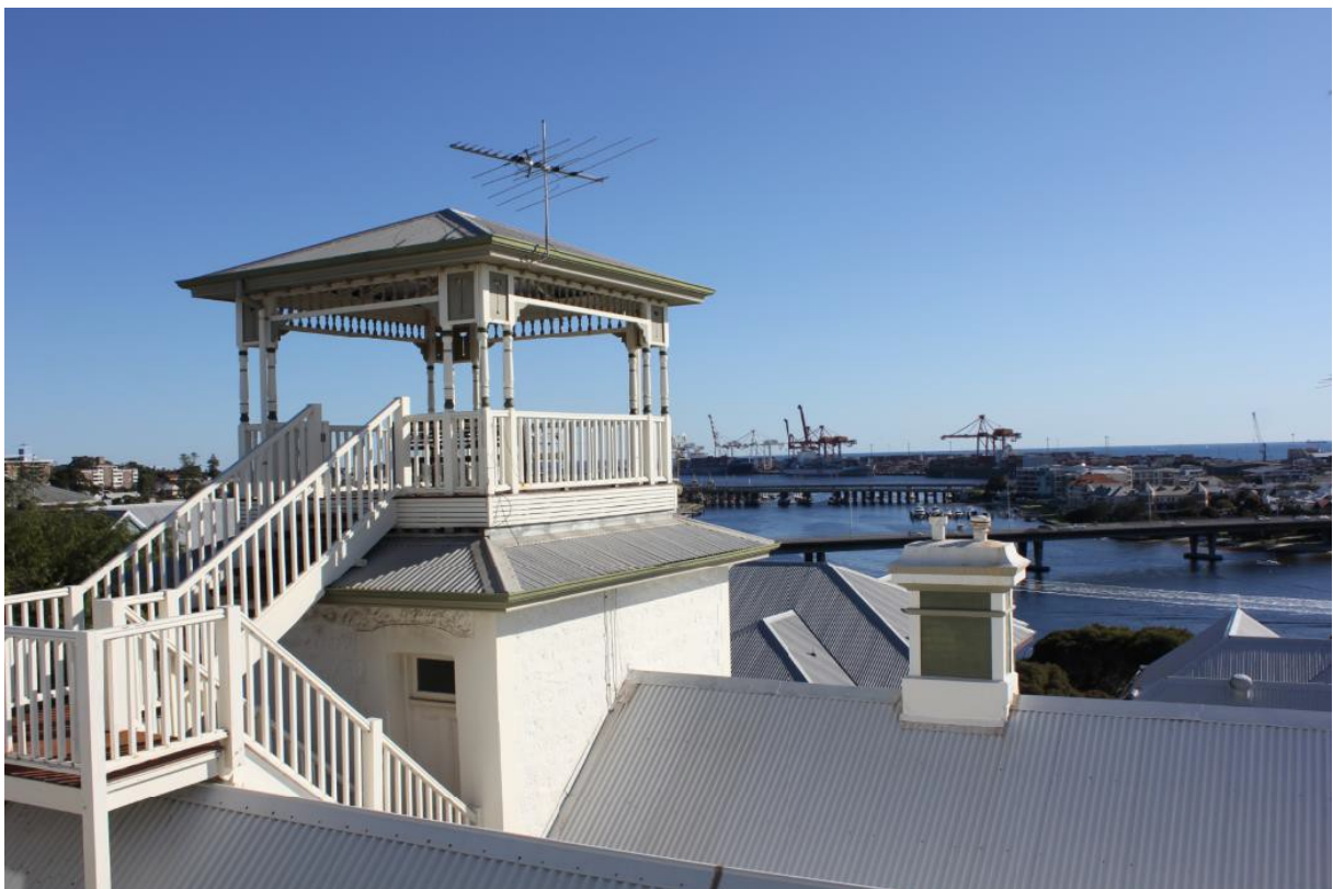
Figure 5. Roofline 10 Bolton Street.
