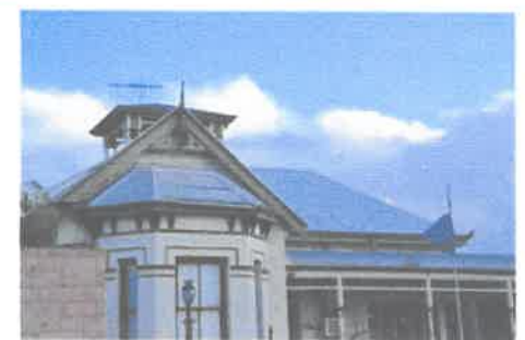
VIEW FROM 9 BOLTON STREET
