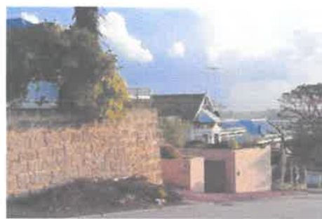
VIEW FROM 5 Bolton Street
