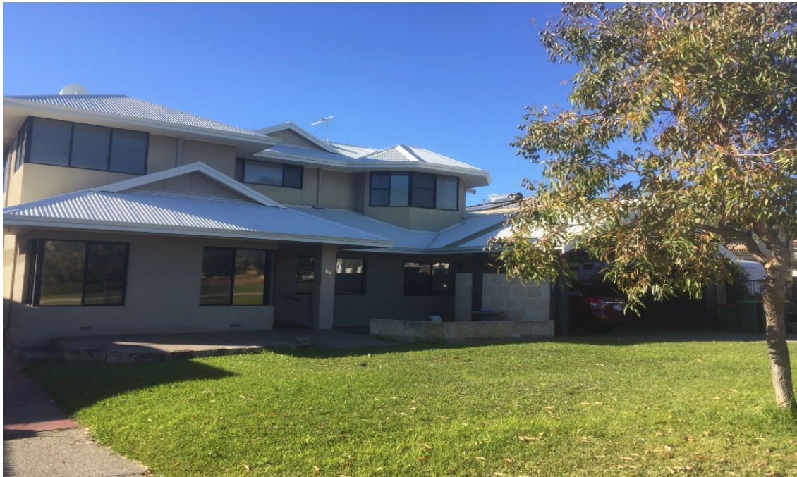
64 A Clayton Street – Photos
