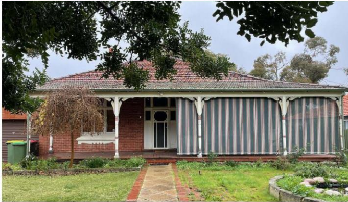
Photograph 1 View from the street. Griffiths Architects July 2022
