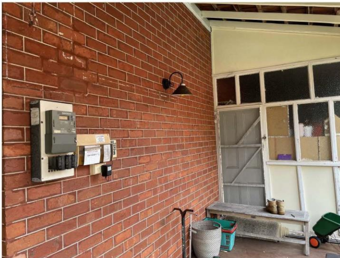
Photograph 3 The east tuck-pointed wall and later verandah sleepout. Griffiths Architects July 2022
