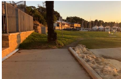
Existing pathway end point
