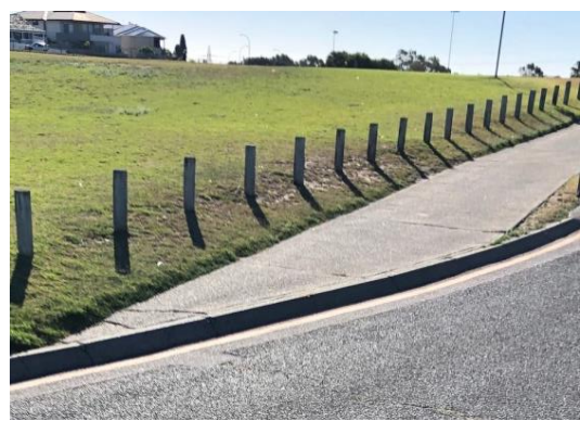
Facing west from triangle - no gutter ramp
