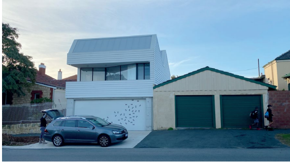
156 George Street - Garage and loft addition (4 houses along from 148 George Street)
