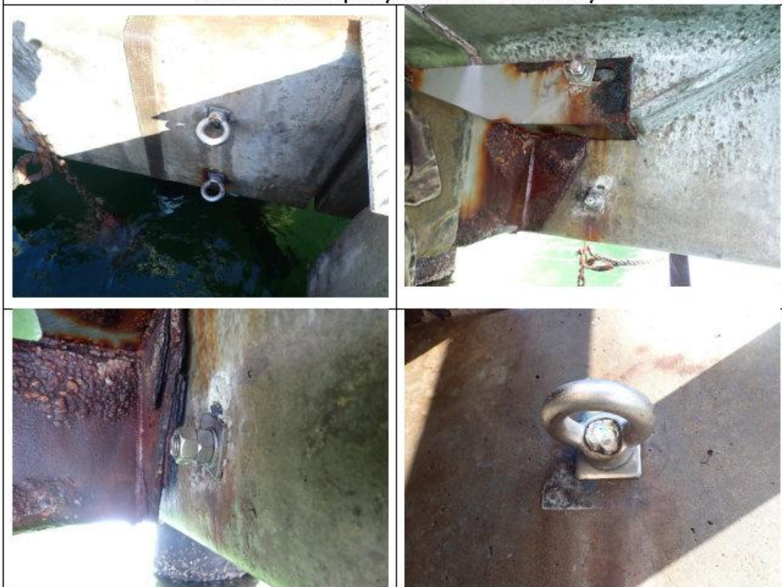
New stainless steel pad eyes installed on Middle Jetty
