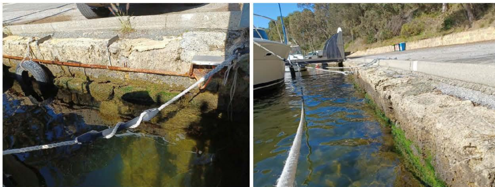
Figure 3.28 Limestone Blockwall
