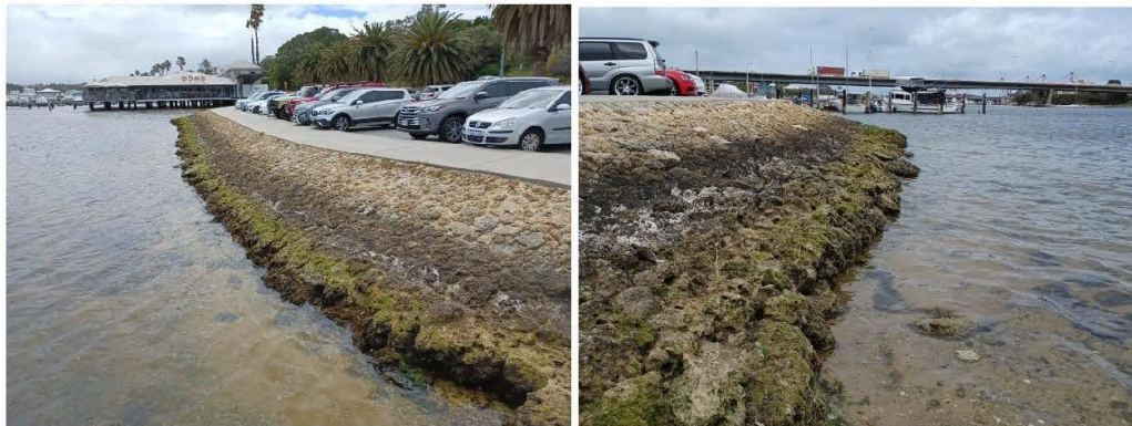
Figure 3.6 Pitched Revetment Looking North (L) & South (R)
