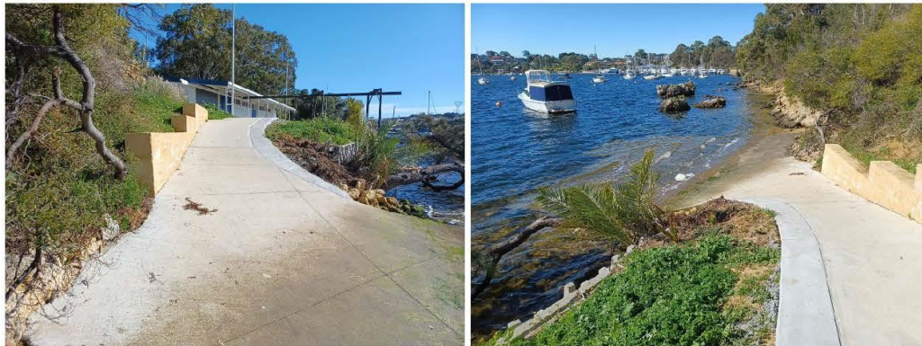
Figure 3.25 Limestone Block Wall & Concrete Apron
