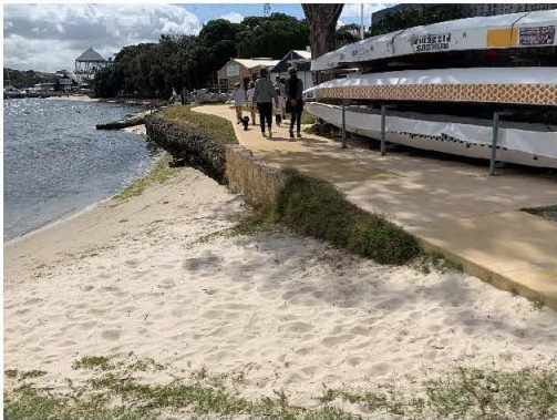
Figure 3.17 Limestone Block Wall
