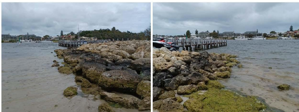
Figure 3.13 Revetment Around Boat Ramp
