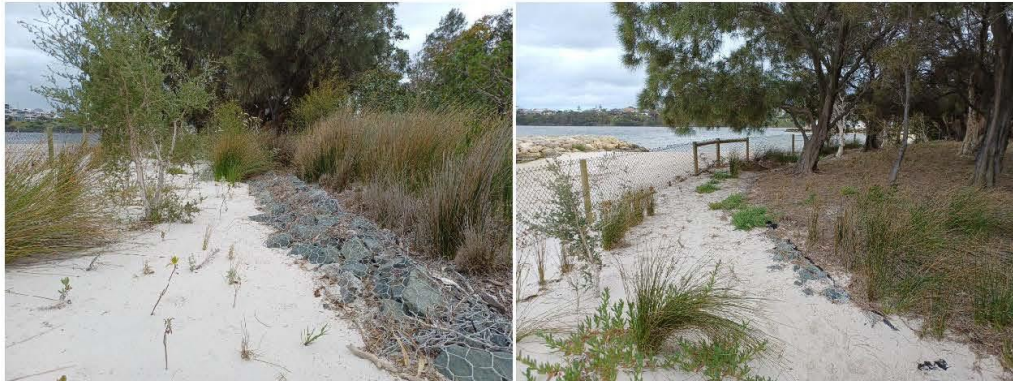
Figure 3.15 Buried Gabion/Reno Mattresses
