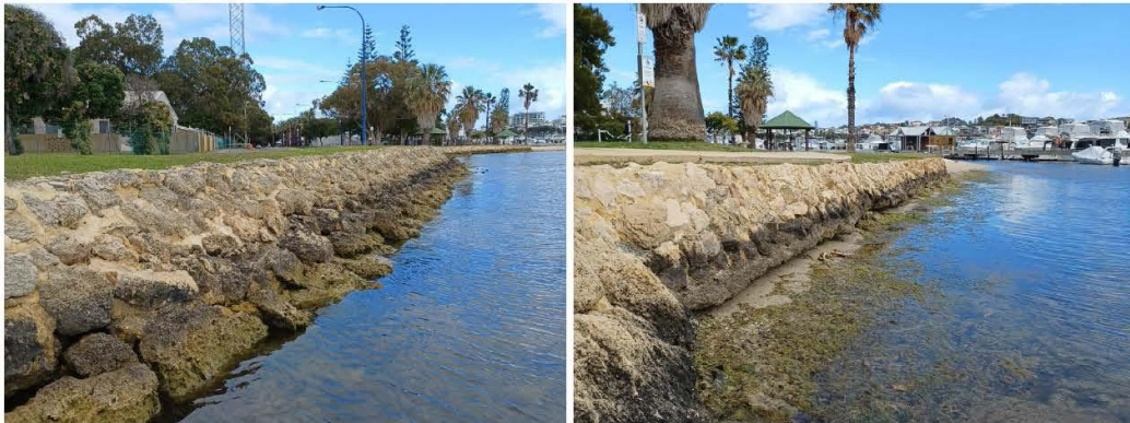
Figure 3.22 Pitched Limestone Revetment
