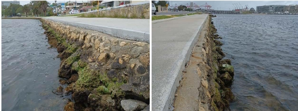
Figure 3.2 J Dolan Park Wall Looking East (L) & Looking West (R)
