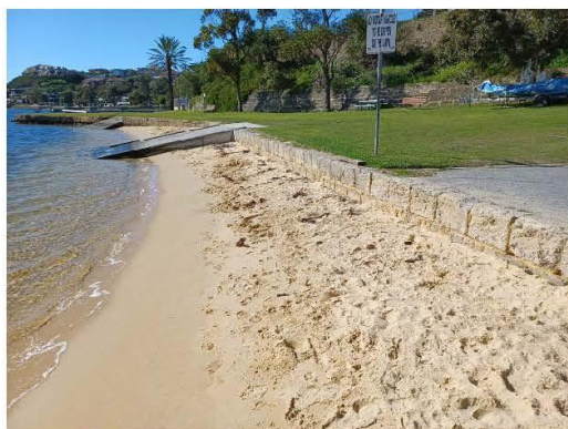
Figure 3.35 Limestone Blockwall
