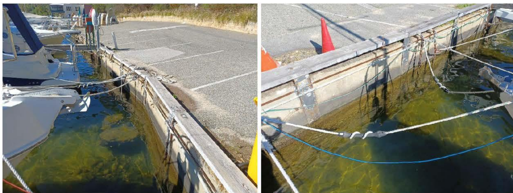
Figure 3.30 Concrete Panel & Steel Pile Wall
