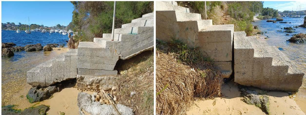
Figure 3.26 Concrete Stair Abutment
