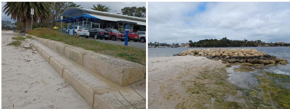
Figure 3.14 Block Wall (L) & Groyne Example (R)
