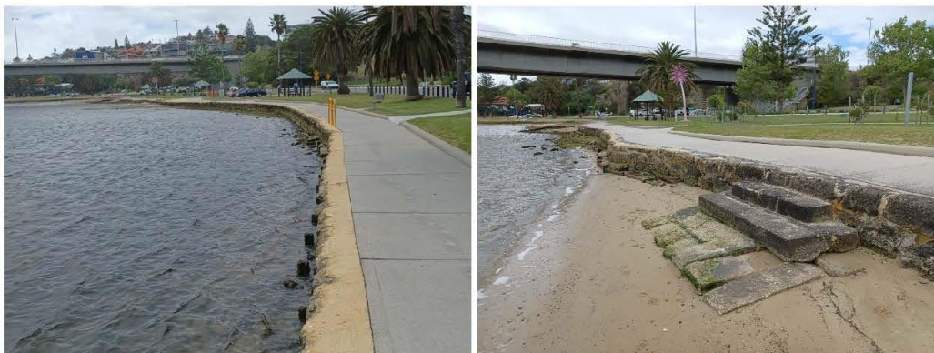
Figure 3.3 Limestone Block Wall (L) & Access Stairs (R)
