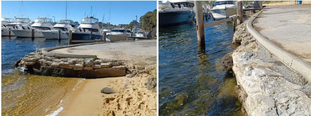
Figure 3.27 Grout Filled Bags
