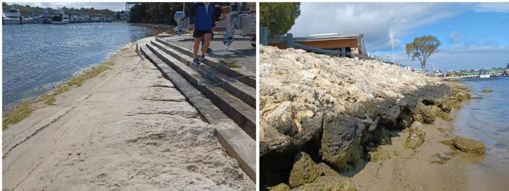
Figure 3.20 Steps (L) & Pitched Revetment (R)
