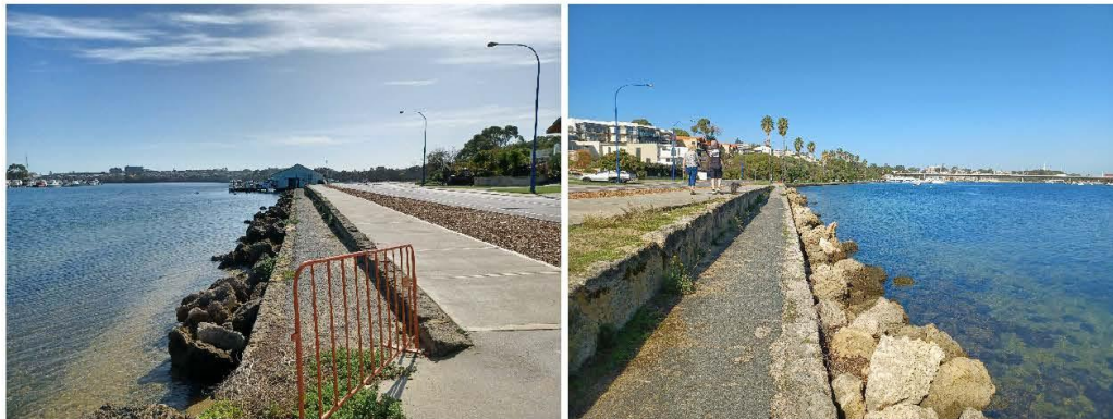
Figure 3.9a Limestone Armour in Front of Vertical Wall
