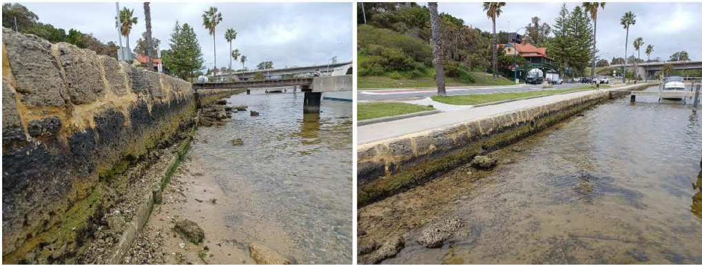
Figure 3.5 Limestone Blockwall with Jetty Abutments
