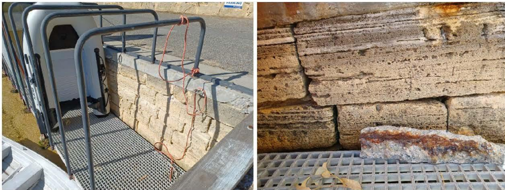
Figure 3.32 Limestone Blockwall with Dinghy Rack
