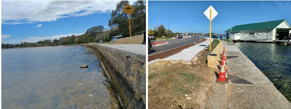
Figure 3.10 Block Wall Section (L) & Settled Path (R)
