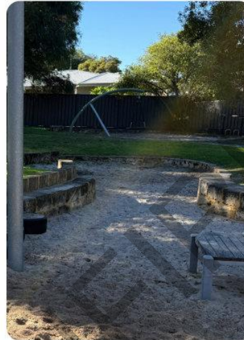
Existing limestone retaining wall
