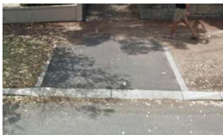
Image 1. Image shows grey concrete footpath priority over driveway and crossover.
