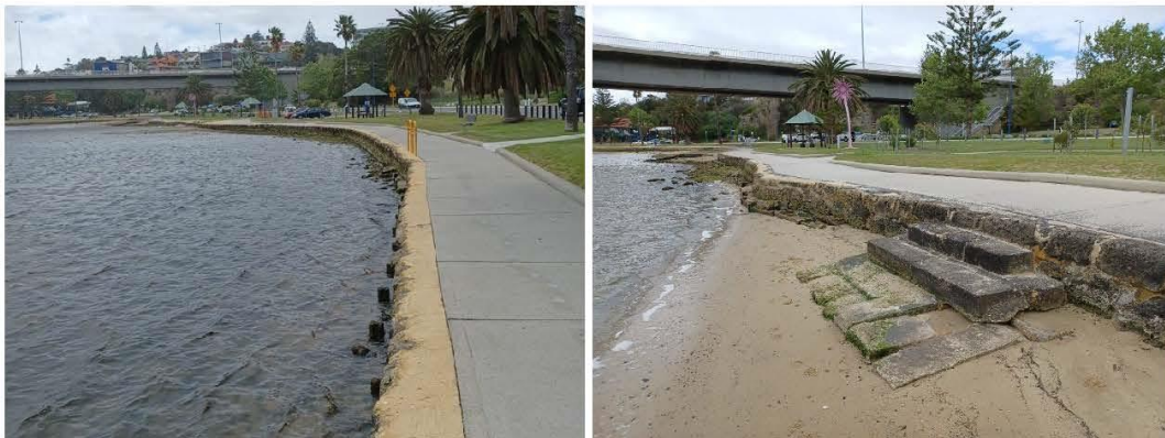
Figure 3.3 Limestone Block Wall (L) & Access Stairs (R)
