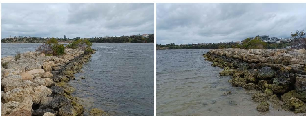
Figure 3.16 Preston Point Groyne
