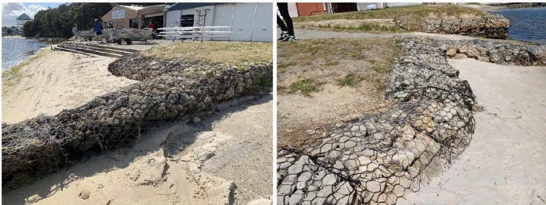
Figure 3.19 Limestone Gabions
