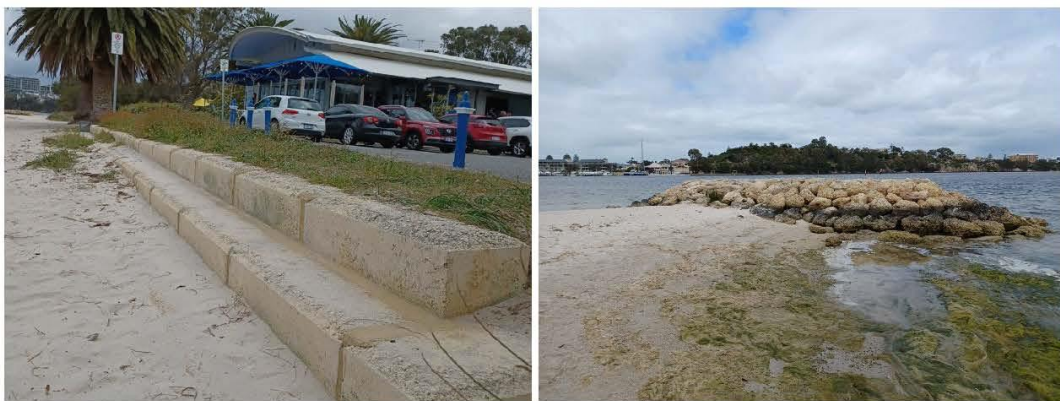
Figure 3.14 Block Wall (L) & Groyne Example (R)
