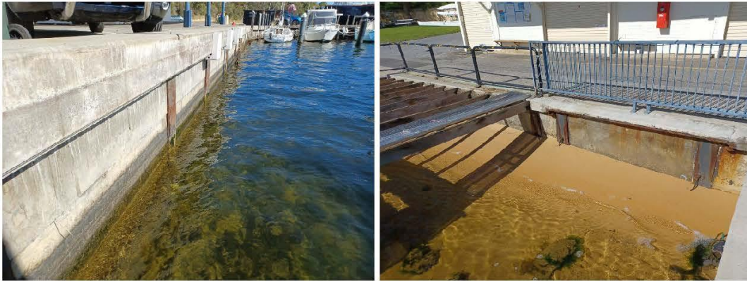
Figure 3.34 Concrete Panel & Steel H-Pile Wall
