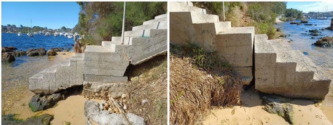
Figure 3.26 Concrete Stair Abutment
