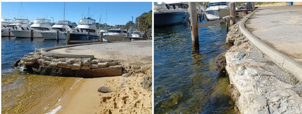
Figure 3.27 Grout Filled Bags
