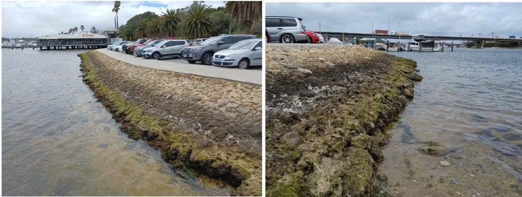
Figure 3.6 Pitched Revetment Looking North (L) & South (R)
