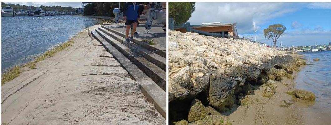
Figure 3.20 Steps (L) & Pitched Revetment (R)
