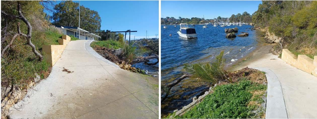
Figure 3.25 Limestone Block Wall & Concrete Apron
