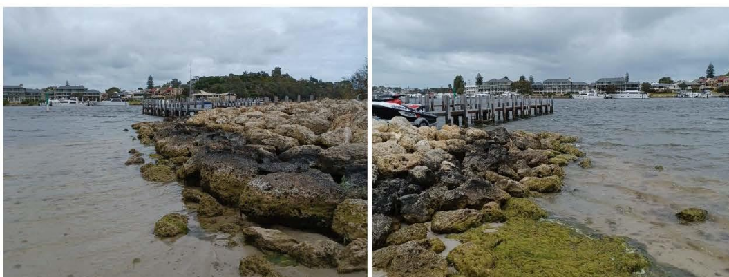
Figure 3.13 Revetment Around Boat Ramp
