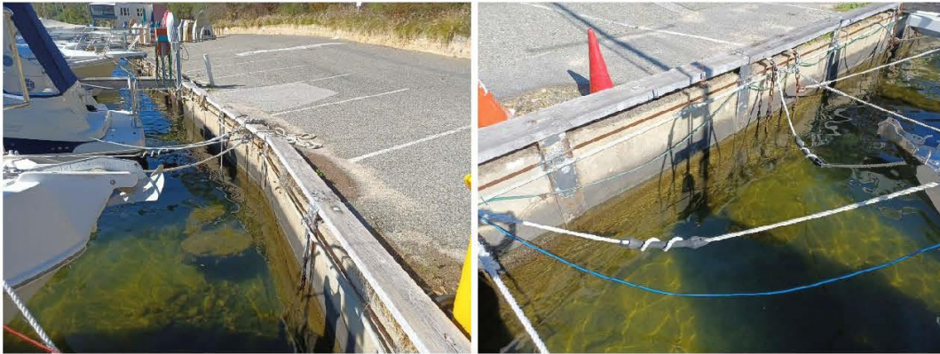
Figure 3.30 Concrete Panel & Steel Pile Wall
