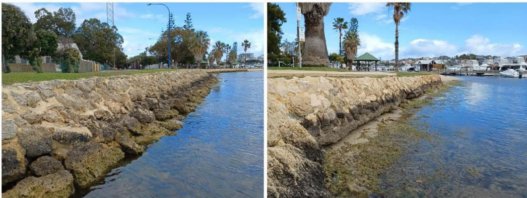
Figure 3.22 Pitched Limestone Revetment
