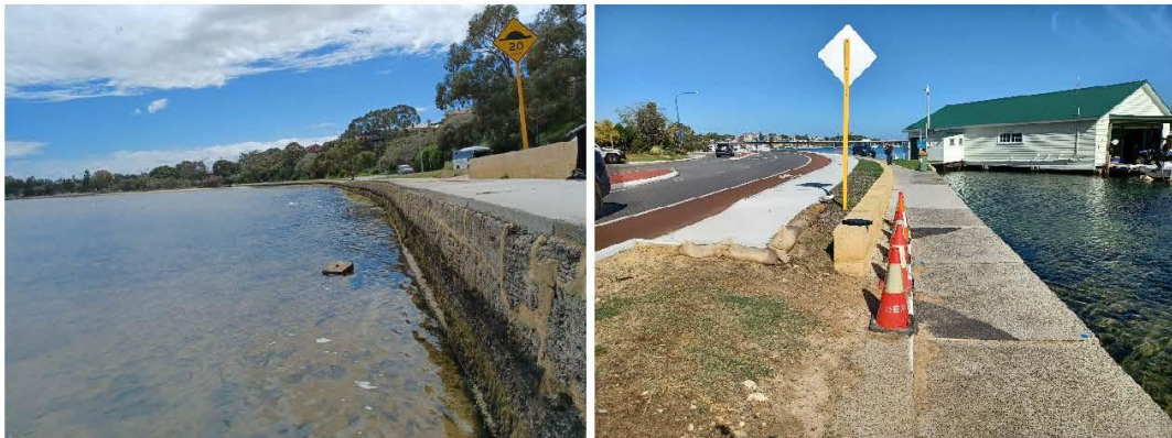
Figure 3.10 Block Wall Section (L) & Settled Path (R)
