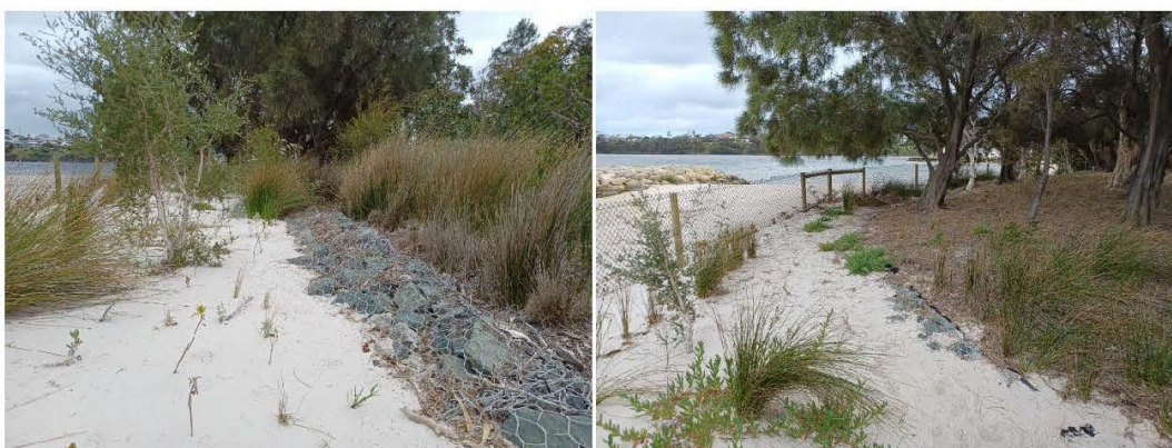
Figure 3.15 Buried Gabion/Reno Mattresses
