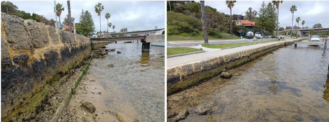
Figure 3.5 Limestone Blockwall with Jetty Abutments
