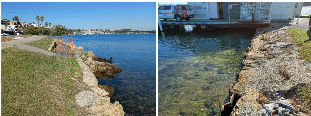
Figure 3.9b Tie In (L) & Sheet Pile Wall (R)
