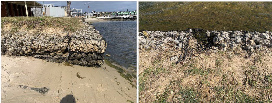
Figure 3.18 Limestone Gabions Rotated (L) & Lost Material (R)
