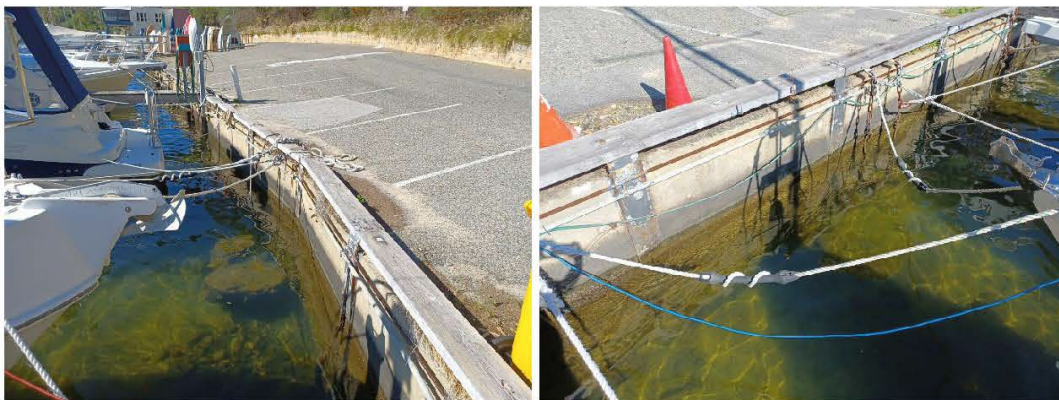
Figure 3.30 Concrete Panel & Steel Pile Wall
