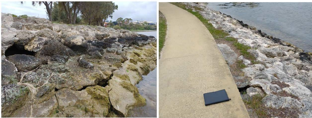
Figure 3.12 Grouted Revetment (L) & Voids Under Path (R)
