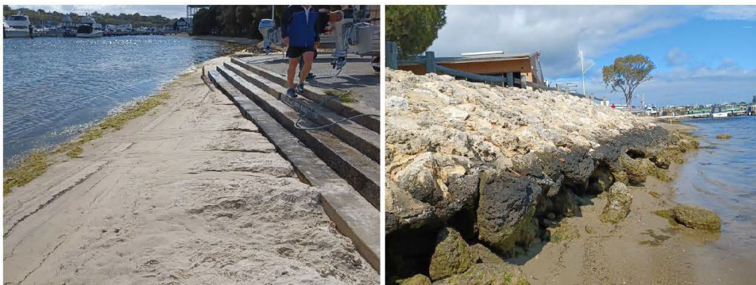
Figure 3.20 Steps (L) & Pitched Revetment (R)
