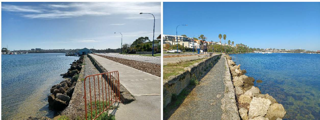
Figure 3.9a Limestone Armour in Front of Vertical Wall
