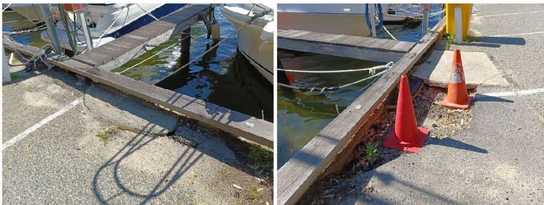
Figure 3.31 Carpark Bitumen Repairs & Settlement
