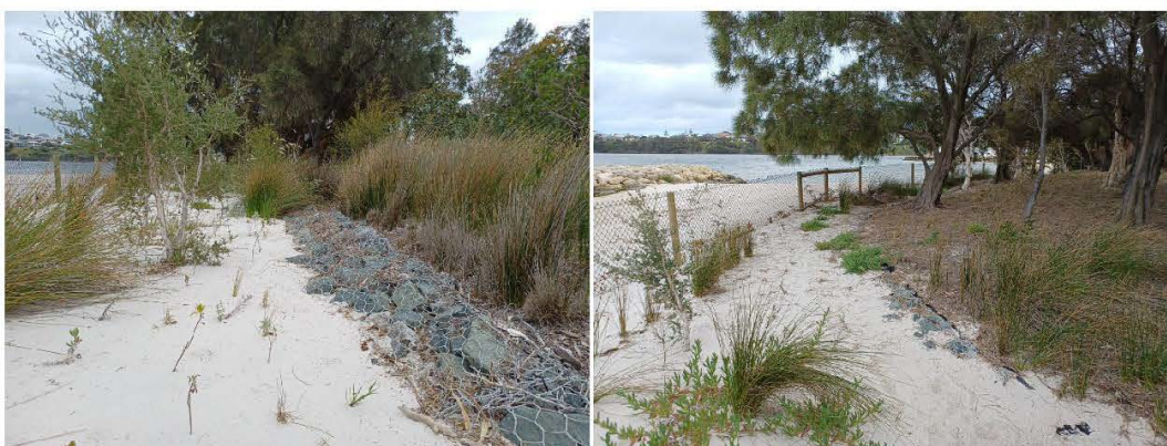
Figure 3.15 Buried Gabion/Reno Mattresses
