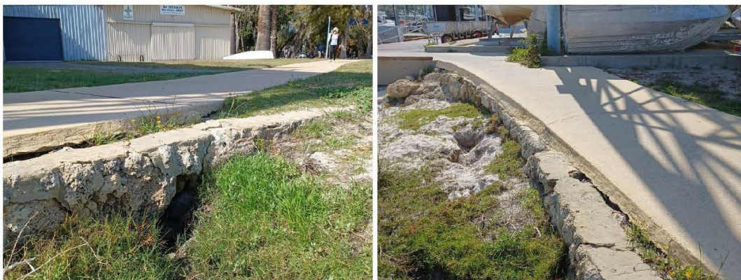
Figure 3.21 Undermined Limestone Block Wall
