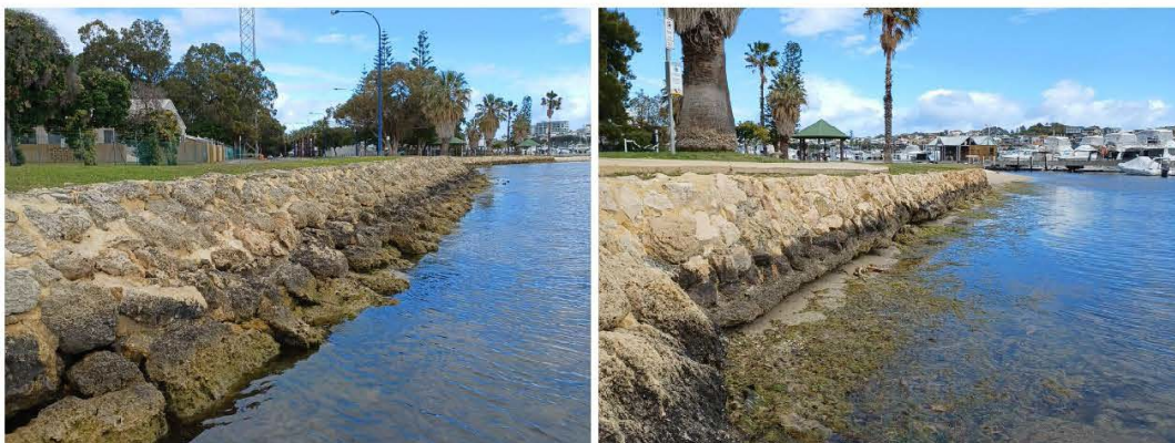
Figure 3.22 Pitched Limestone Revetment
