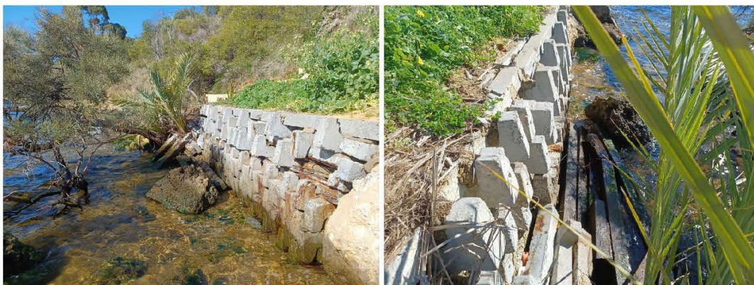
Figure 3.24 Deteriorated Crib Wall
