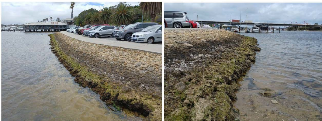
Figure 3.6 Pitched Revetment Looking North (L) & South (R)
