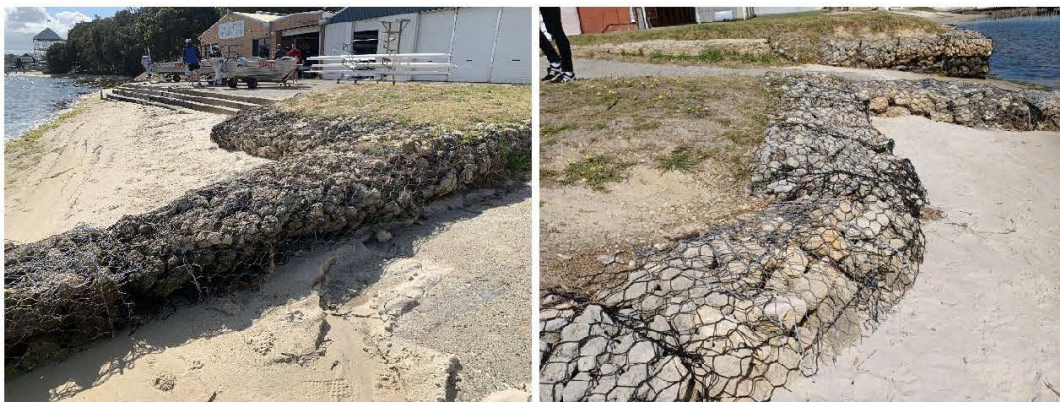
Figure 3.19 Limestone Gabions
