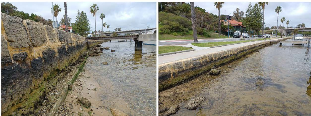
Figure 3.5 Limestone Blockwall with Jetty Abutments
