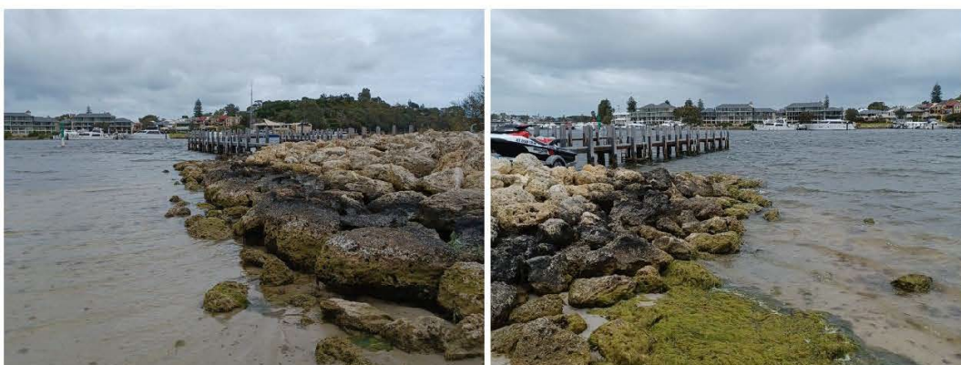
Figure 3.13 Revetment Around Boat Ramp
