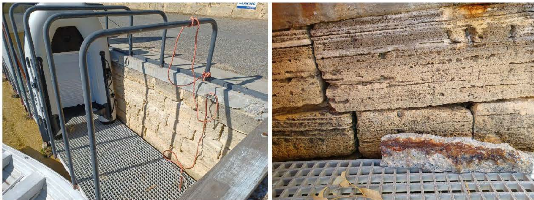
Figure 3.32 Limestone Blockwall with Dinghy Rack
