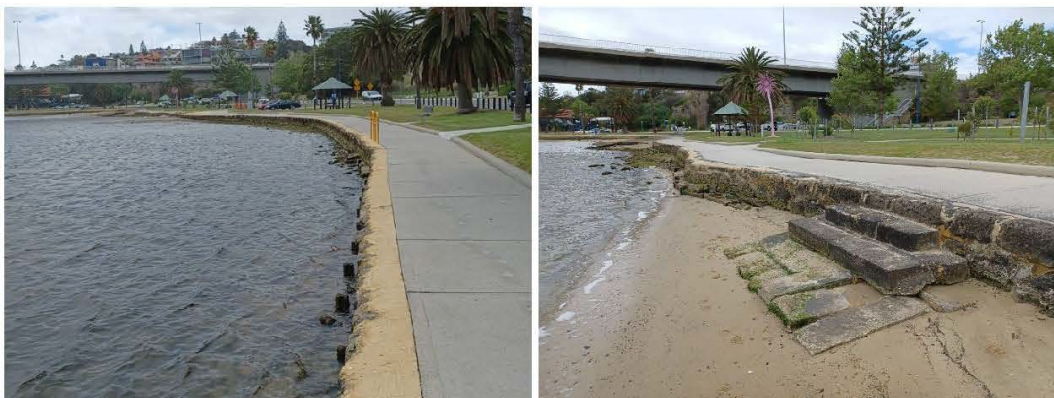
Figure 3.3 Limestone Block Wall (L) & Access Stairs (R)
