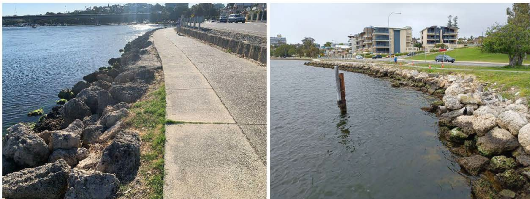
Figure 3.1 Path Behind Revetment (L) & Overtopping Damage (R)
