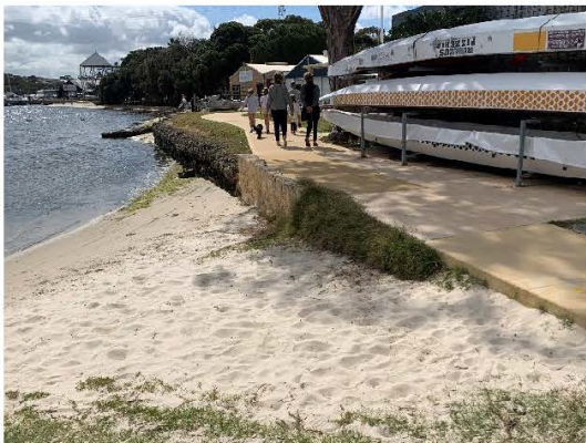
Figure 3.17 Limestone Block Wall
