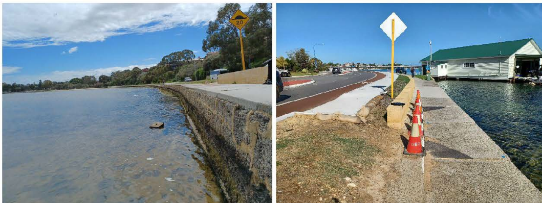
Figure 3.10 Block Wall Section (L) & Settled Path (R)
