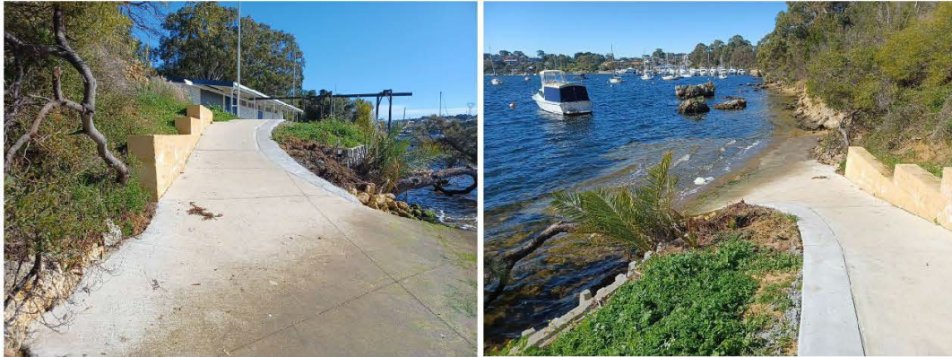
Figure 3.25 Limestone Block Wall & Concrete Apron
