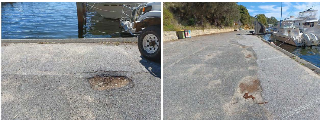
Figure 3.29 Carpark Pot Holes & Repairs
