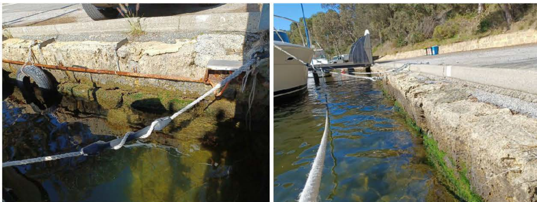
Figure 3.28 Limestone Blockwall
