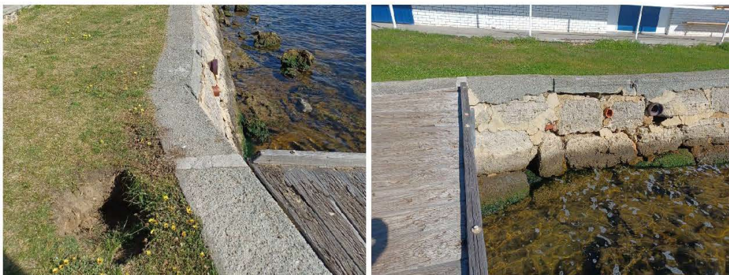
Figure 3.23 Deteriorated Limestone Block Wall
