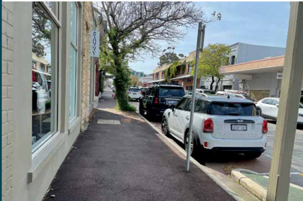
Upgraded footpaths on George Street
