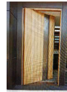
Entrance door with vertical timber slats
