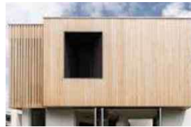
Vertical timber slats in porch area
