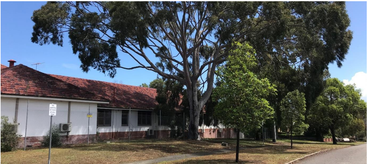
Photograph 10 – Existing Woodside Hospital maternity wing on the subject site (Fortescue Street frontage).
