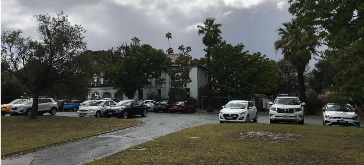
Photograph 3 – Existing Woodside Hospital building viewed from the south west (Dalgety Street).
