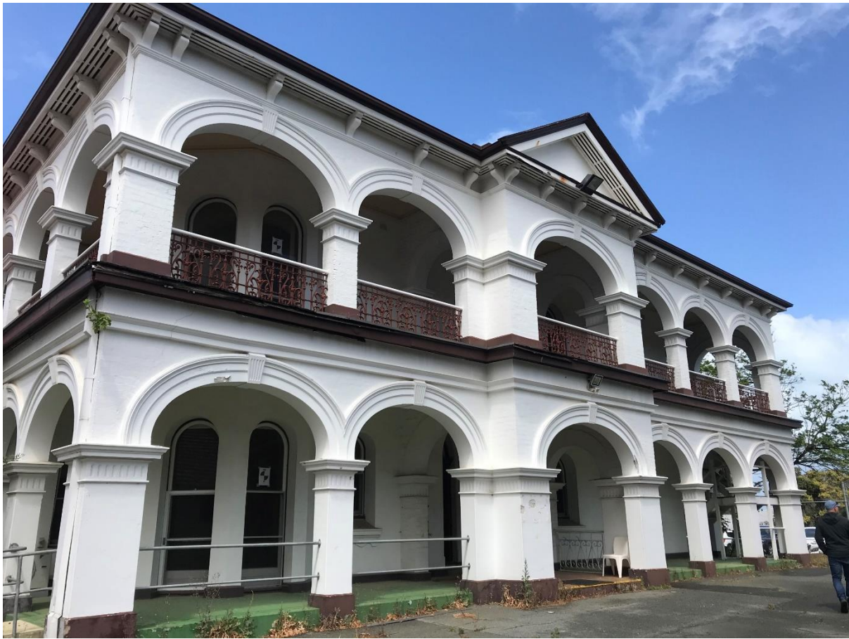
Photograph 1 – Existing Woodside Hospital building on the subject site, western elevation (Dalgety Street frontage).
