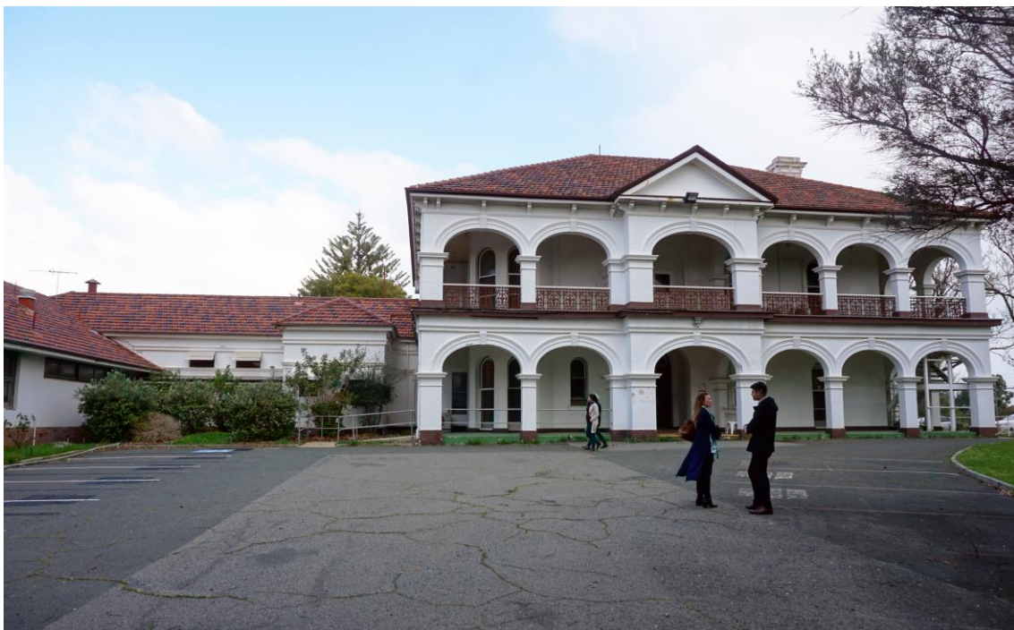
Photo 03 North elevation of Woodside House and former ballroom, cloakroom/ hospital wing conversion.
