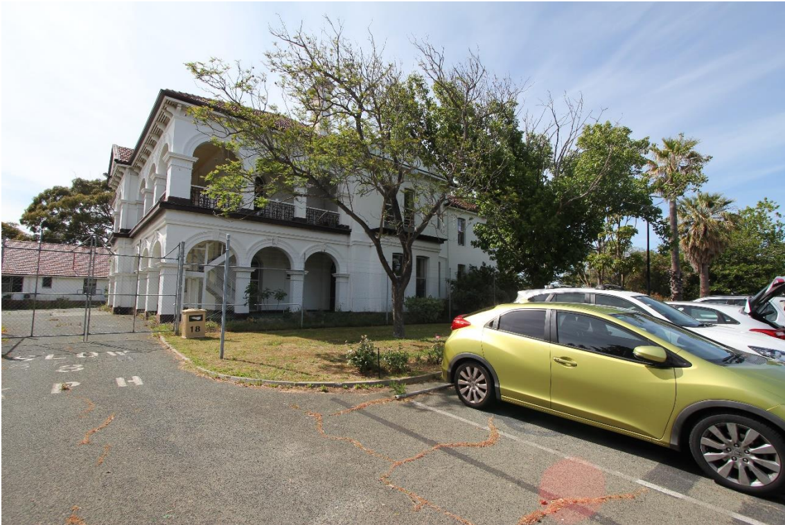
Photo 04 West elevation of Woodside House from west carpark. The servants quarters and kitchen to the right were built as a separate phase.
