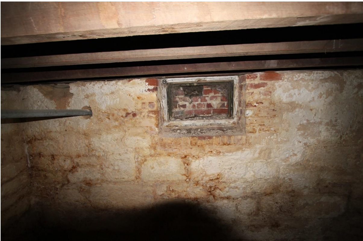
Photo 07 Cellar discovered under former kitchen, to south west of Woodside house.
