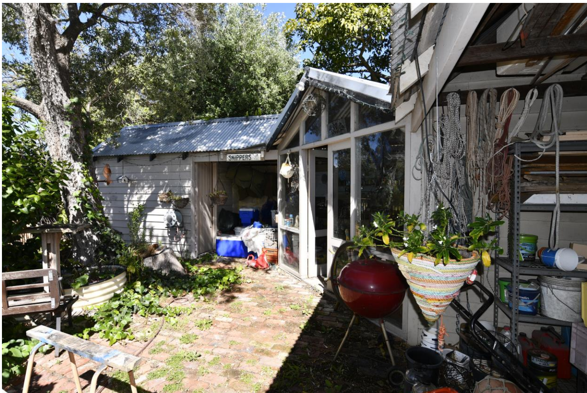
Photo 29 Latter addition timber shed with central glazing and corrugated iron roof.
