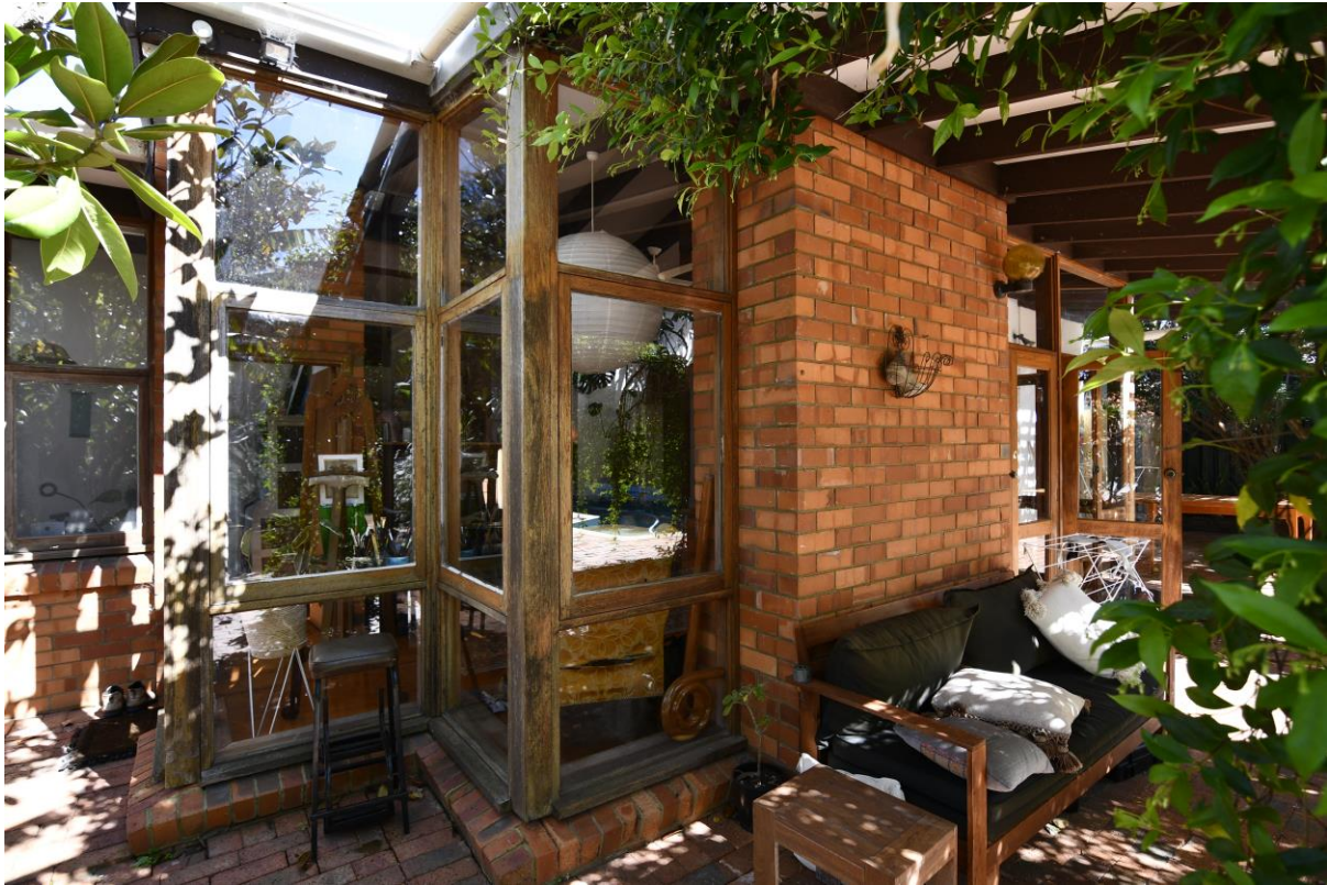
Photo 14 North elevation of 26 Dalgety. The rear addition is constructed of brick with timber framed windows.
