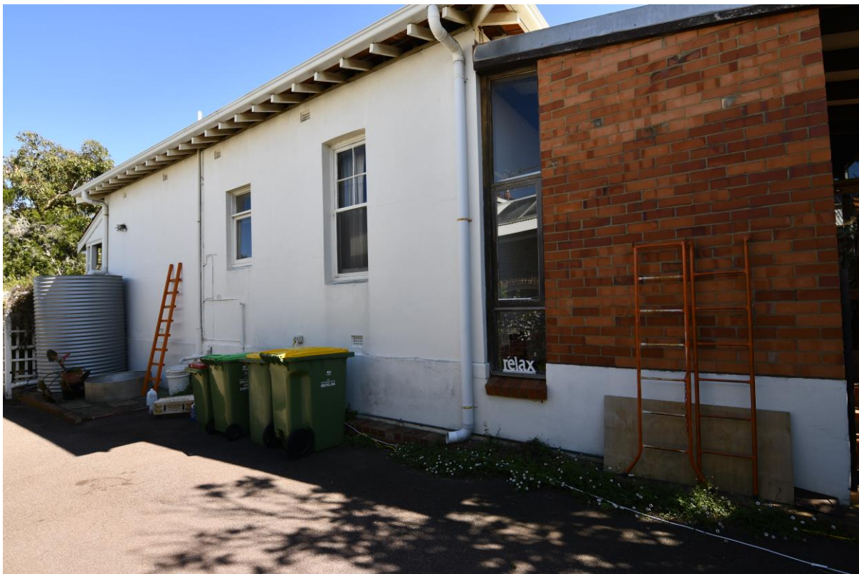
Photo 11 The original south wall to the house has been rendered.
