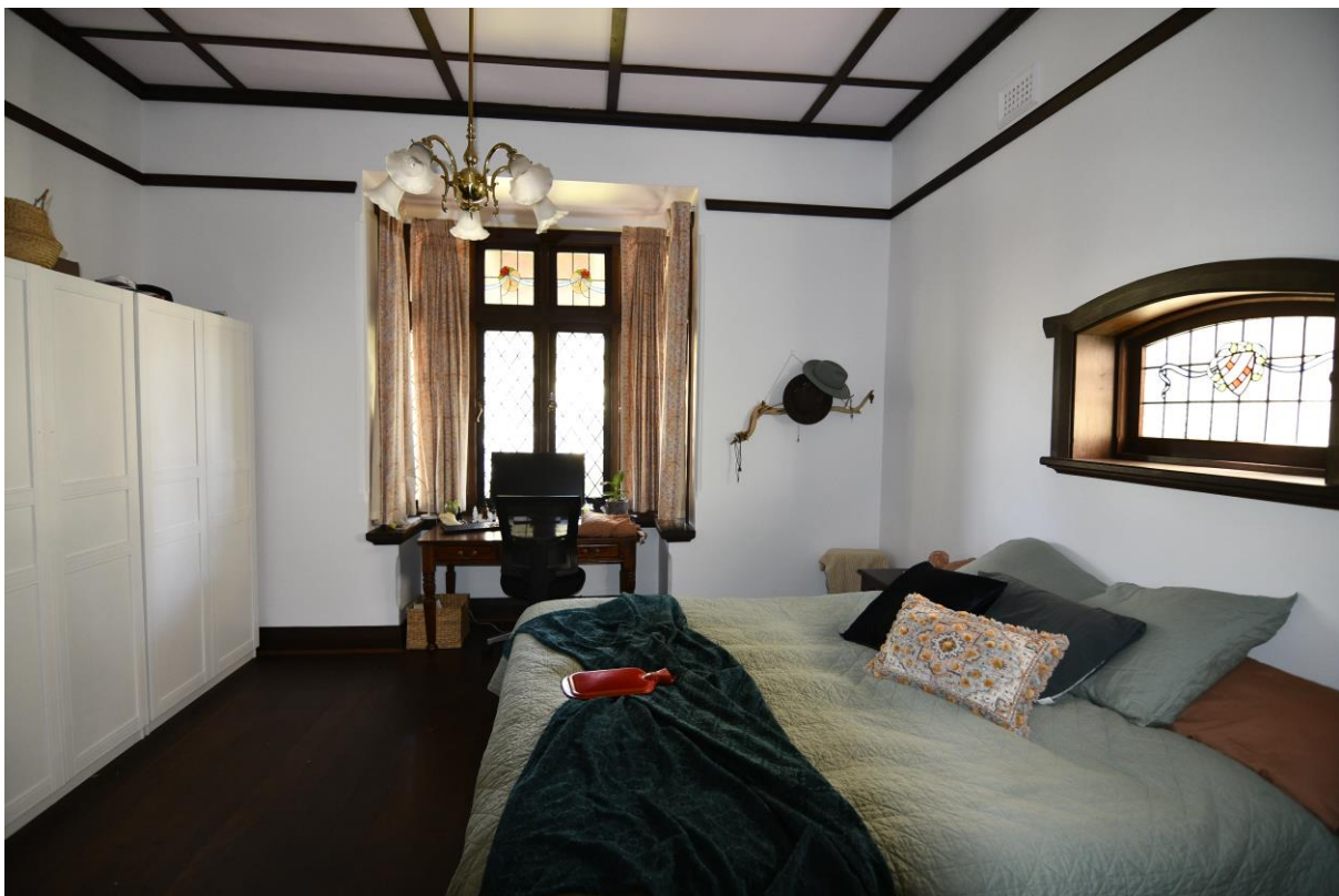
Photo 17 View of Bedroom 2 with lead light glazing in a diamond pattern and motif leadlight fanlights bay window to the front and arched lead light window to the north. Stained timber battens on the ceiling show signs of sagging.
