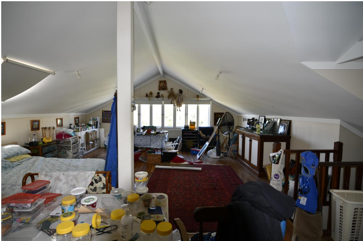
Photo 27 View of the 1990's attic extension, staircase is non-compliant with today's standards.
