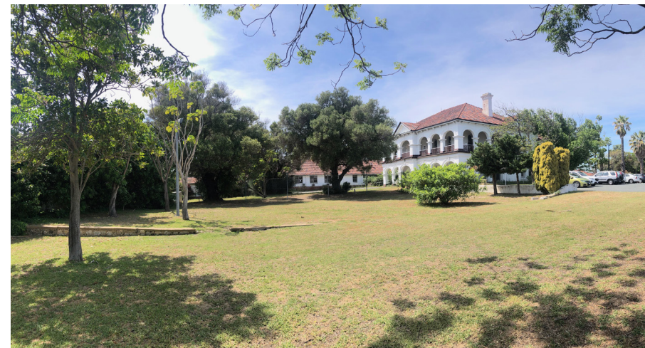
EXISTING NORTH WEST VIEW OF SITE
