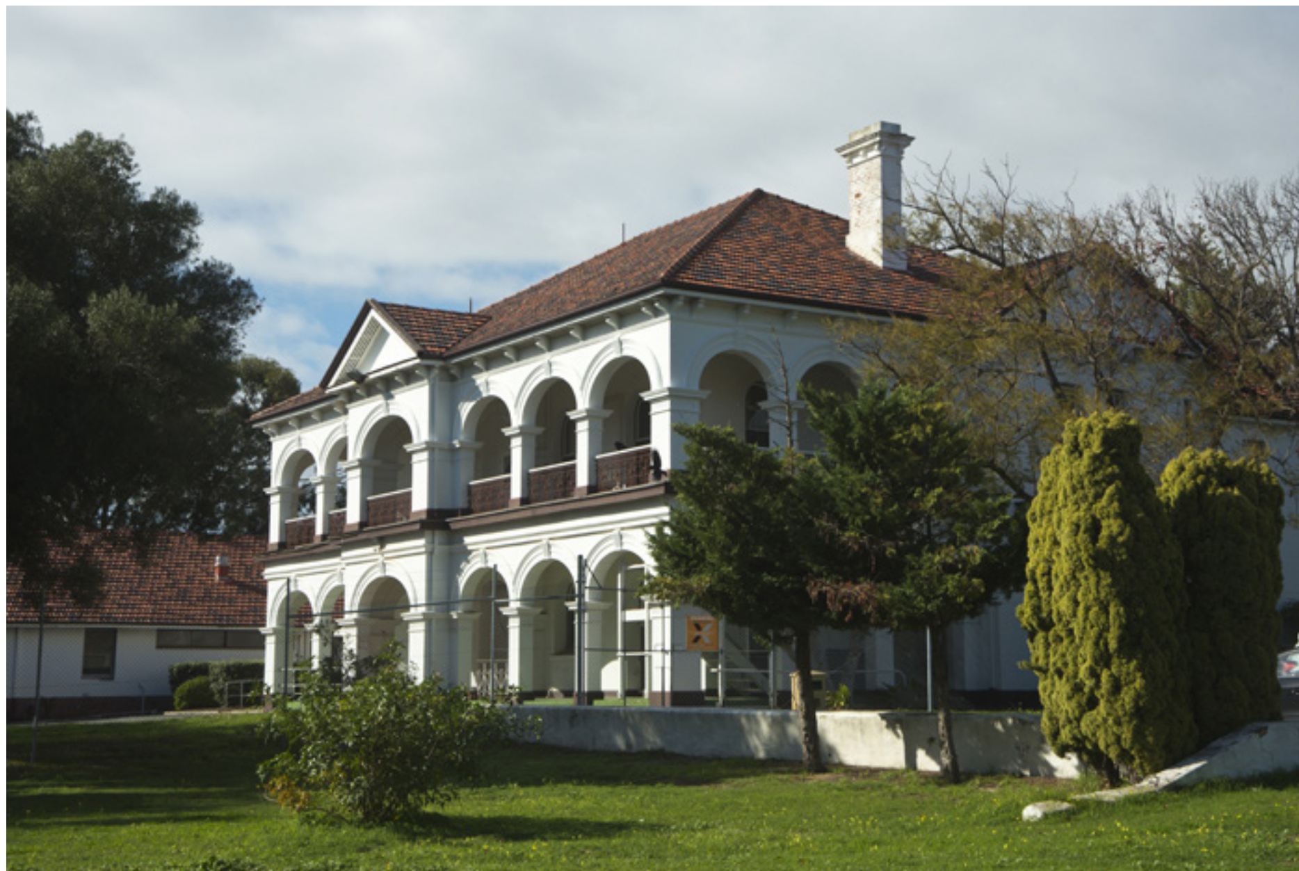
EXISTING NORTH WEST VIEW OF WOODSIDE HOUSE
