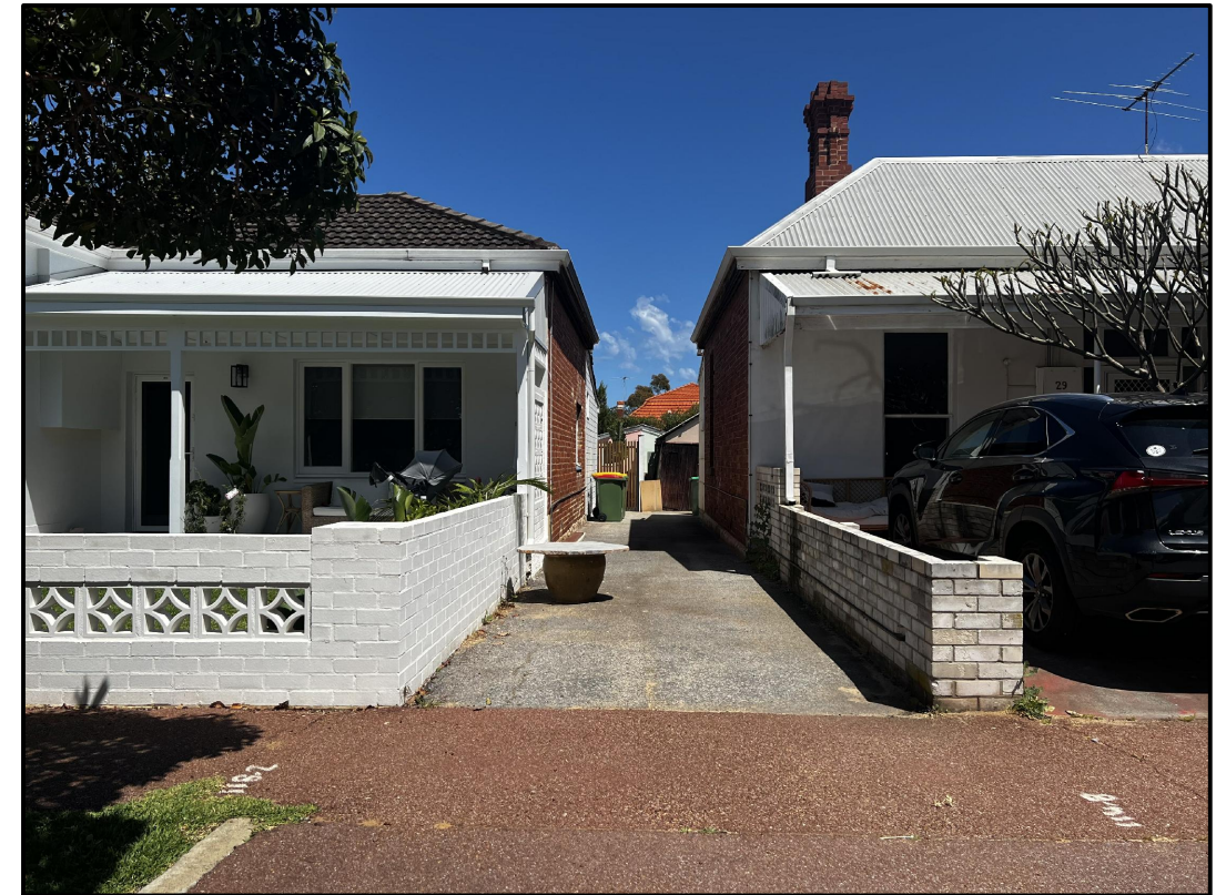
STREETSCAPE CLOSE UP - CURRENT
