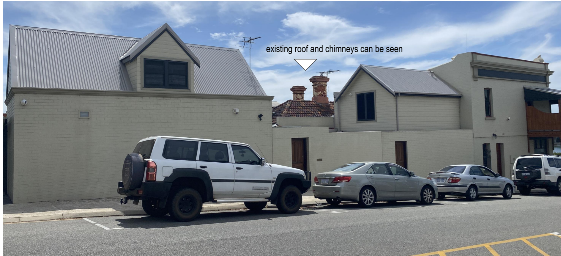
east elevation of home is obstructed by 55 Canning Highway - street image supplied in lieu of elevation
