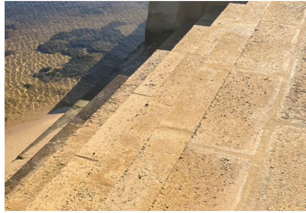
Reconstituted limestone blockwork to be used in terraced steps
