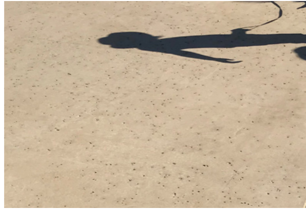
Plaza paving with concrete in sand/ limestone colour
