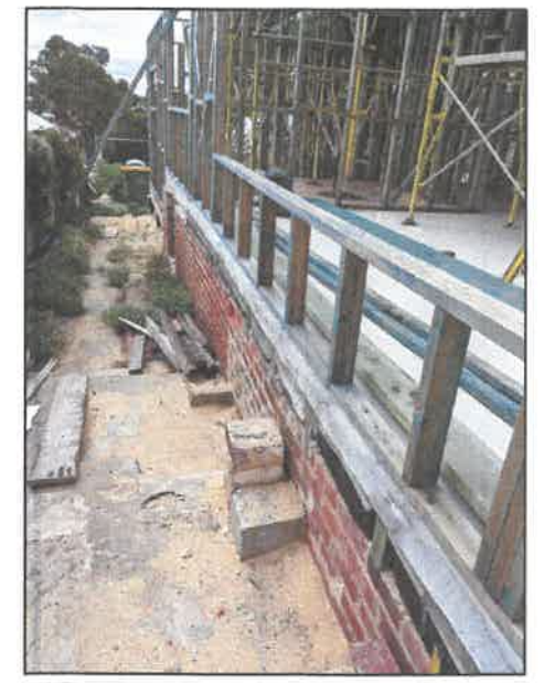
VIEW OF EXISTING HEIGHTS 2
