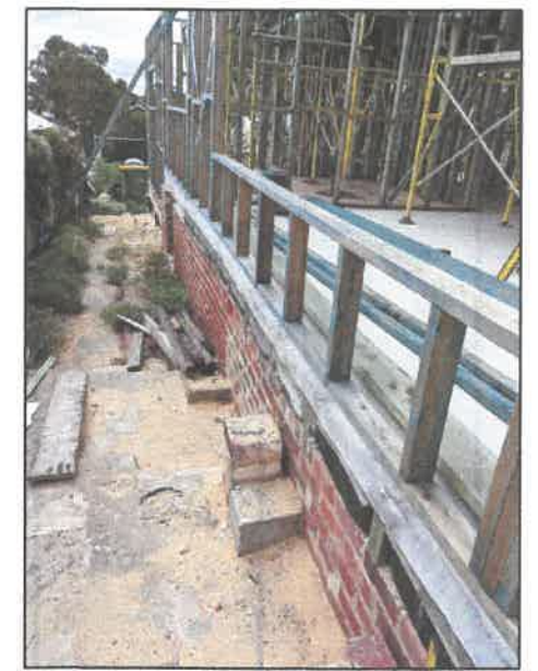
VIEW OF EXISTING HEIGHTS 2
