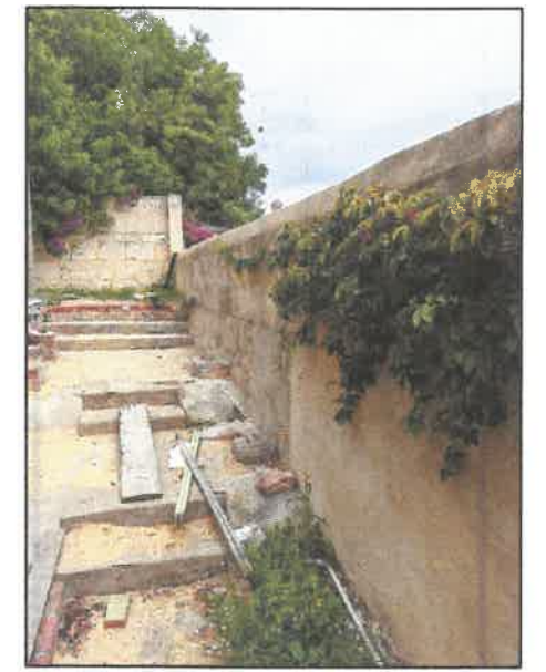
VIEW OF EXISTING HEIGHTS 4
