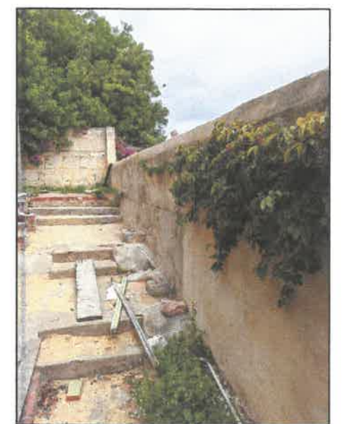
VIEW OF EXISTING HEIGHTS 4
