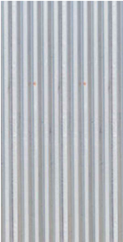
CORRUGATED IRON ROOFING
