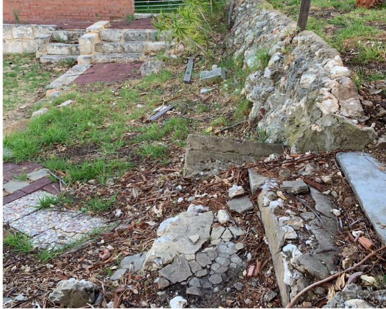
Existing Retaining Wall and Steps (Proposed to be demolished)
