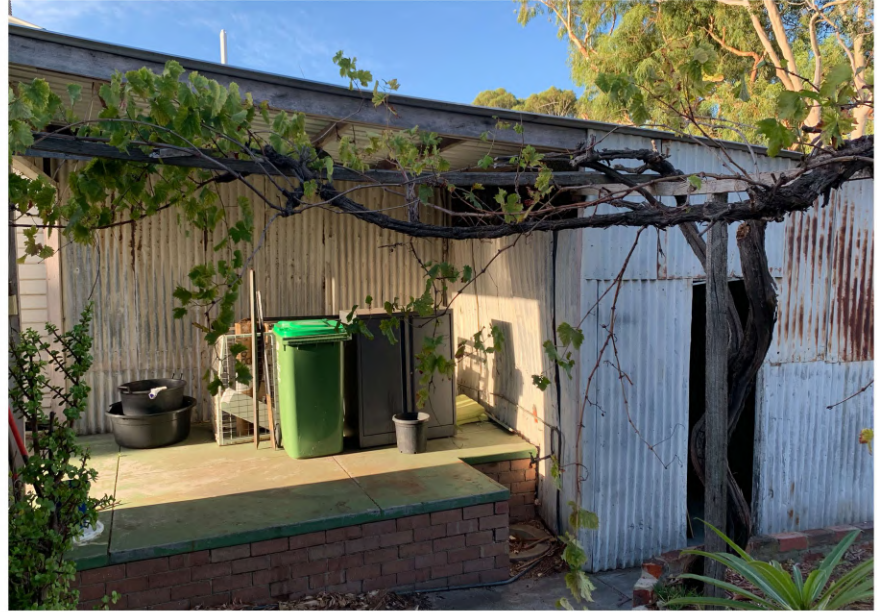
Existing Metal Sheds (Proposed to be demolished)
