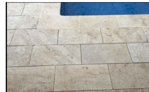
TRAVERTINE PAVING LAID IN STRETCHER BOND PATTERNS AS PER PICTURE ABOVE PAVING AREAS: TOTAL BELOW 228sqm EXCLUDING OFFCUTS - FRONT PORCH AND SIDE OF HOUSE DOWN TO LAUNDRY - SIDE OF GARAGE AND STORE INCLUDING STAIRCASE DOWN - LOWER GROUND FLOOR SITTING AREA AND RAMP DOWN TO POOL - POOL AREA INCLUDING POOL AREA STAIRCASE
