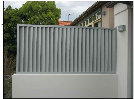
MINIMUM 1600mm HIGH BALCONY ALUMINIUM OR SIMILAR PRIVACY SCREEN - CAN BE A SOLID BRICK WALL OR FROSTED GLASS SCREEN MINIMUM 1.6m HIGH
