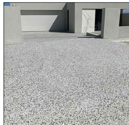
CONCRETE DRIVEWAY AND CROSSOVER WASHED AGGREGATE LIMECRETE SALT AND PEPPER OR SIMILAR - APPROX 110gsm
