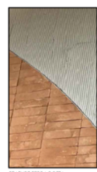
FEATURE TERRACOTTA BRICKWORK.
