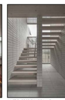
WHITE FACE BRICKWORK AND CONCRETE STAIRS.
