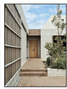
WHITE BRICK OR BLOCK WORK EXTERIOR WALLS. TERRACOTTA PAVING TO WALKWAYS. FEATURE ENTRY DOOR AND TIMBER SCREENS. FEATURE PLANTING TO ATRIUMS AND GARDEN BEDS.
