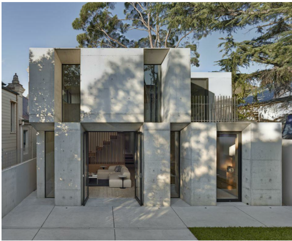
INISITU CONCRETE WALL: OFF-FORM FINISH
