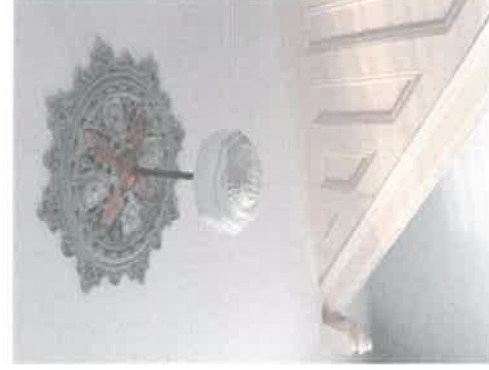
timber paneling and trims to existing stairwell
