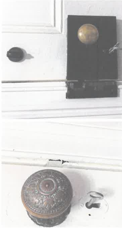
Original Doors + Door Hardware
