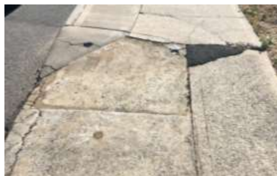
Cracked pavement repaired but uneven
