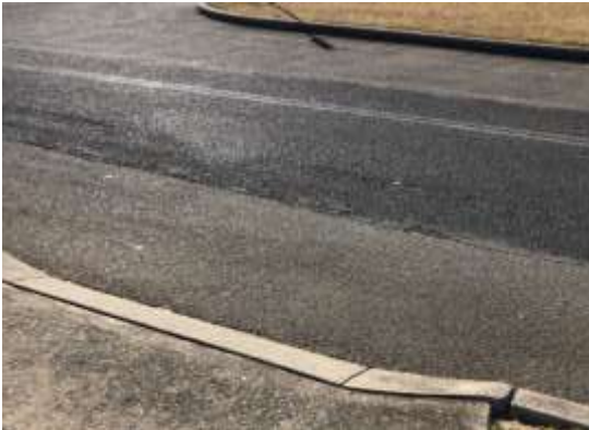
Median strip –no gutter ramp opposite
