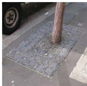
↻ Steel angle edging with granite sett and bonded stone aggregate infill
