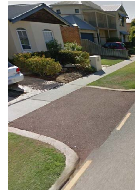
Image 15. Image shows red asphalt crossover and grey concrete footpath priority over crossover. Source: www.nearmap.com.au, street view. Accessed 2019.
