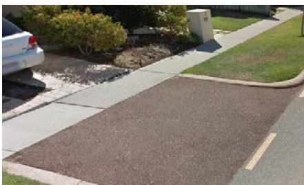
Image 1. Image shows red asphalt crossover and grey concrete footpath priority over driveway and crossover.
