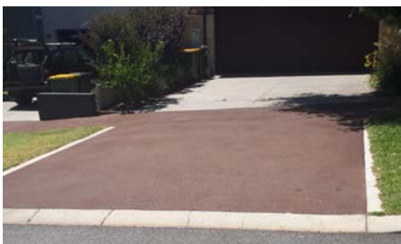
Image 1. Image shows red asphalt footpath and crossover.
