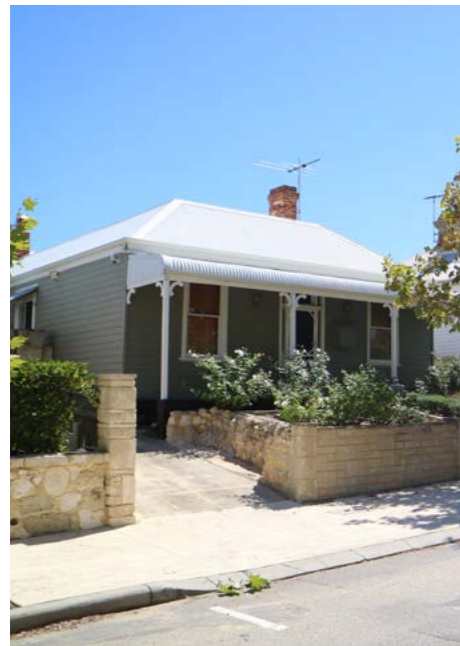
Image 8. Image shows limecrete footpath priority over residential driveway. Source: UDLA.
