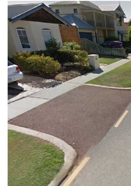
Image 15. Image shows red asphalt crossover and grey concrete footpath priority over crossover. Source: www.nearmap.com.au, street view. Accessed 2019.
