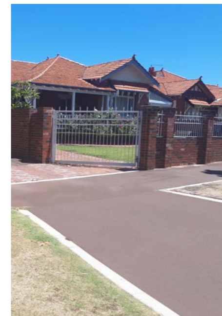
Image 9. Image shows red asphalt footpath priority over residential driveway. Source: UDLA.
