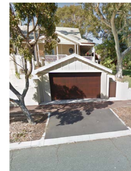
Image 13. Image shows red asphalt footpath priority over residential driveway. Source: www.nearmap.com.au, street view. Accessed 2019.
